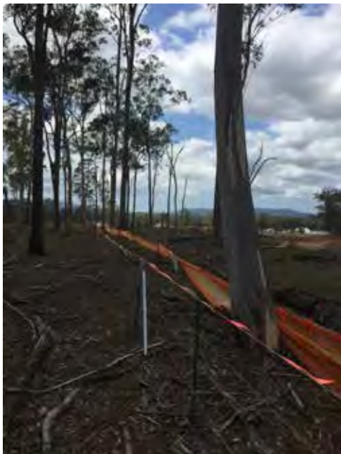
Photo 15. There were approximately 5 trees growing on the road reserve that were not included in the report.
