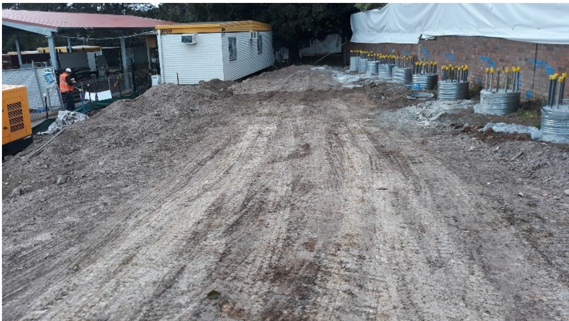
Looking across the Grid 12 area at the Penshurst Public School at completion of visual walkover inspection on 2 August 2019
