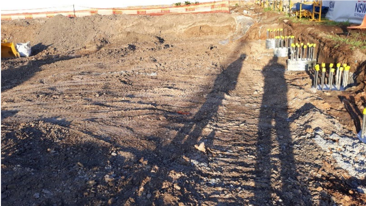
Looking across the Grid 4 and 6 areas at the Penshurst Public School at completion of visual walkover inspection on 5 August 2019
