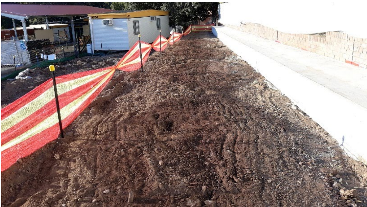
Looking across the Grid 12 area at the Penshurst Public School at completion of visual walkover inspection on 13 August 2019
