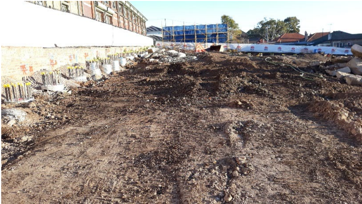
Looking across the Grid 8 area at the Penshurst Public School at completion of visual walkover inspection on 6 August 2019
