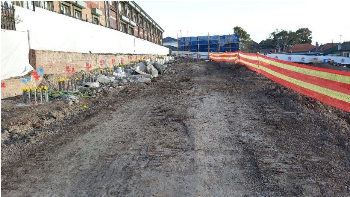
Looking across the Grid 8 area at the Penshurst Public School at completion of visual walkover inspection on 5 August 2019
