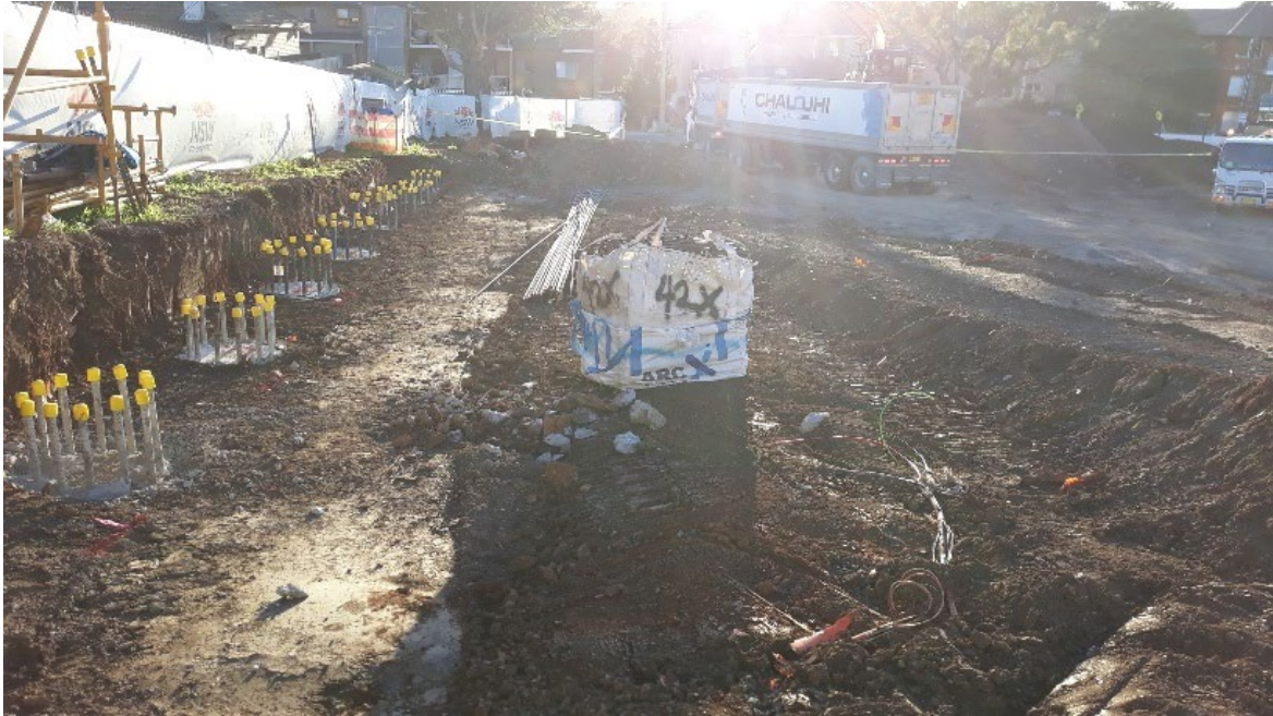
Looking across the Grid 4 and 6 areas at the Penshurst Public School at completion of visual walkover inspection on 9 August 2019
