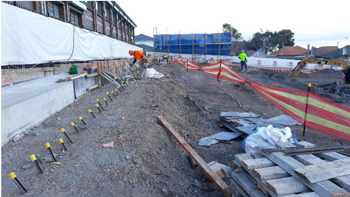
Looking across the Grid 8 area at the Penshurst Public School at completion of visual walkover inspection on 12 August 2019
