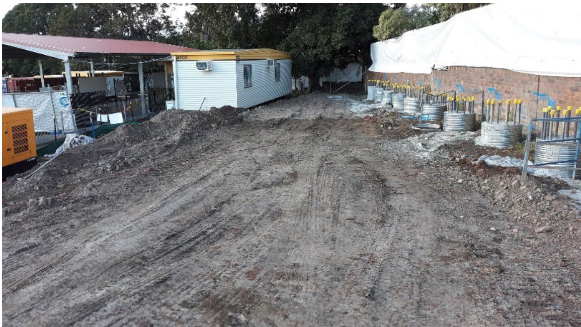
Looking across the Grid 12 area at the Penshurst Public School at completion of visual walkover inspection on 1 August 2019
