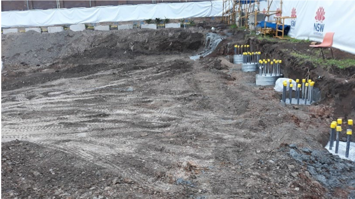
Looking across the Grid 4 and 6 areas at the Penshurst Public School at completion of visual walkover inspection on 2 August 2019
