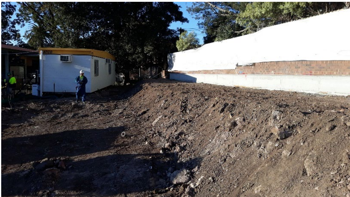
Looking across the Grid 12 area at the Penshurst Public School at completion of visual walkover inspection on 14 August 2019
