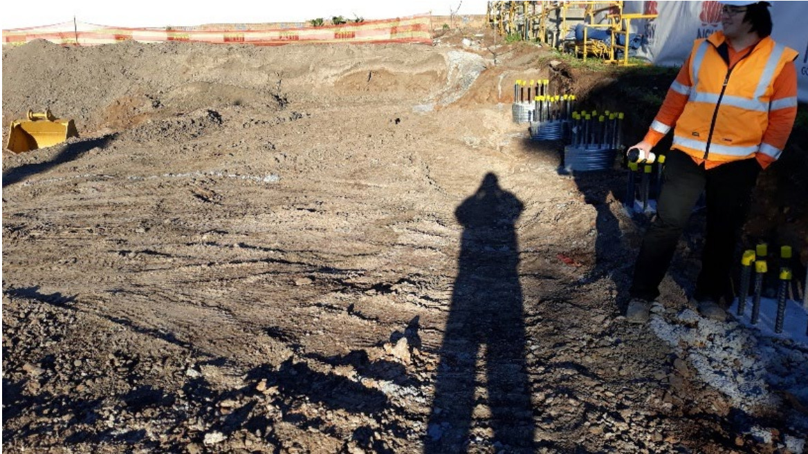
Looking across the Grid 4 and 6 areas at the Penshurst Public School at completion of visual walkover inspection on 6 August 2019
