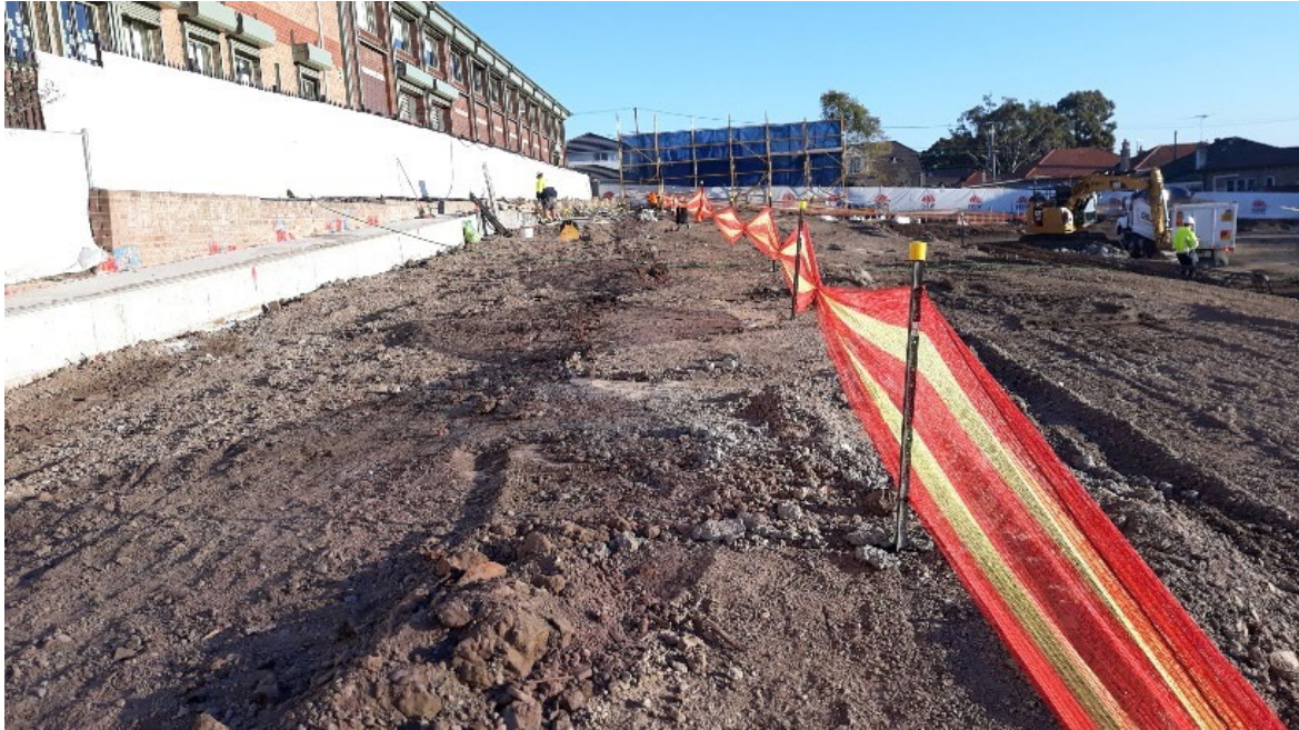
Looking across the Grid 8 area at the Penshurst Public School at completion of visual walkover inspection on 14 August 2019
