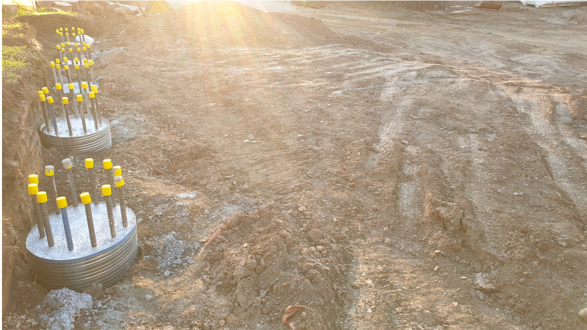
Looking across the Grid 4 and 6 areas at the Penshurst Public School at completion of visual walkover inspection on 7 August 2019
