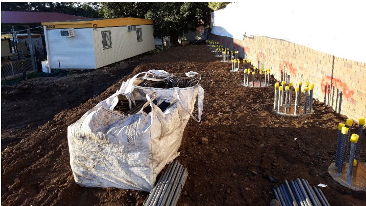
Looking across the Grid 12 area at the Penshurst Public School at completion of visual walkover inspection on 6 August 2019
