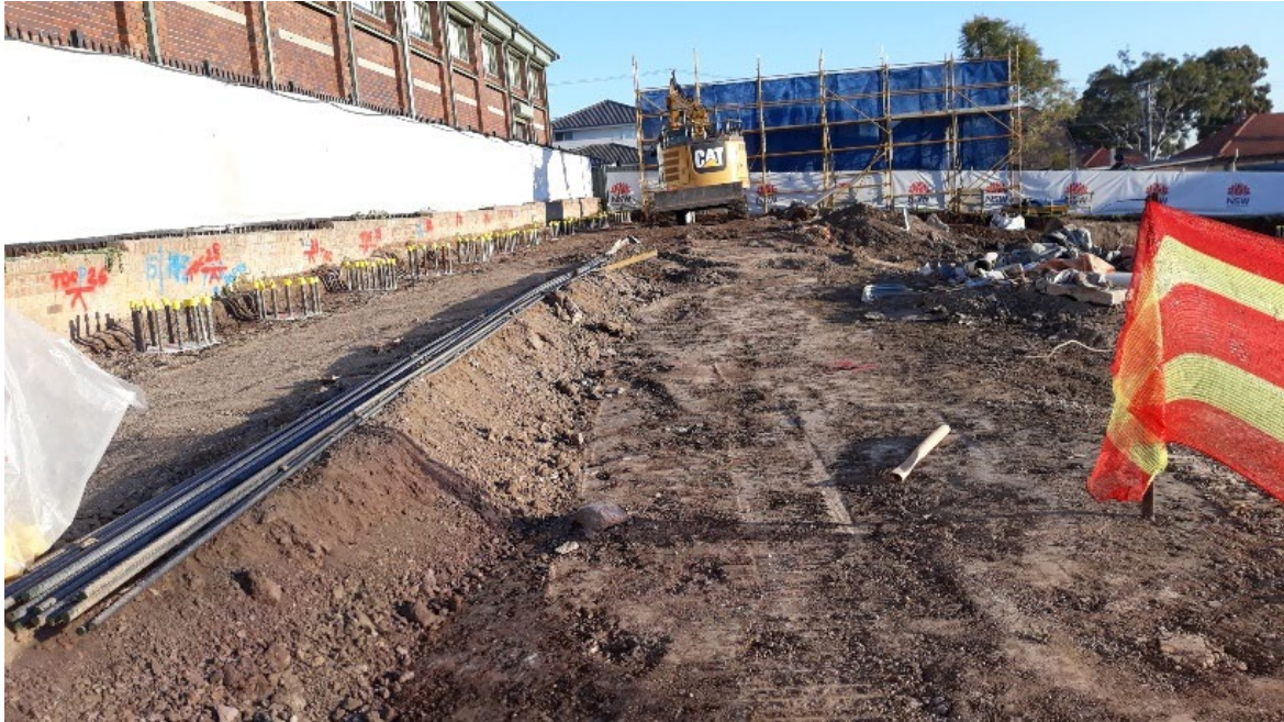
Looking across the Grid 8 area at the Penshurst Public School at completion of visual walkover inspection on 8 August 2019
