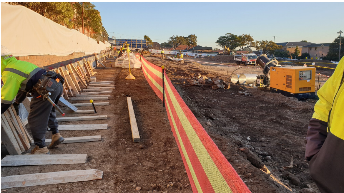
Looking across the Grid 12 area at the Penshurst Public School at completion of visual walkover inspection on 7 August 2019
