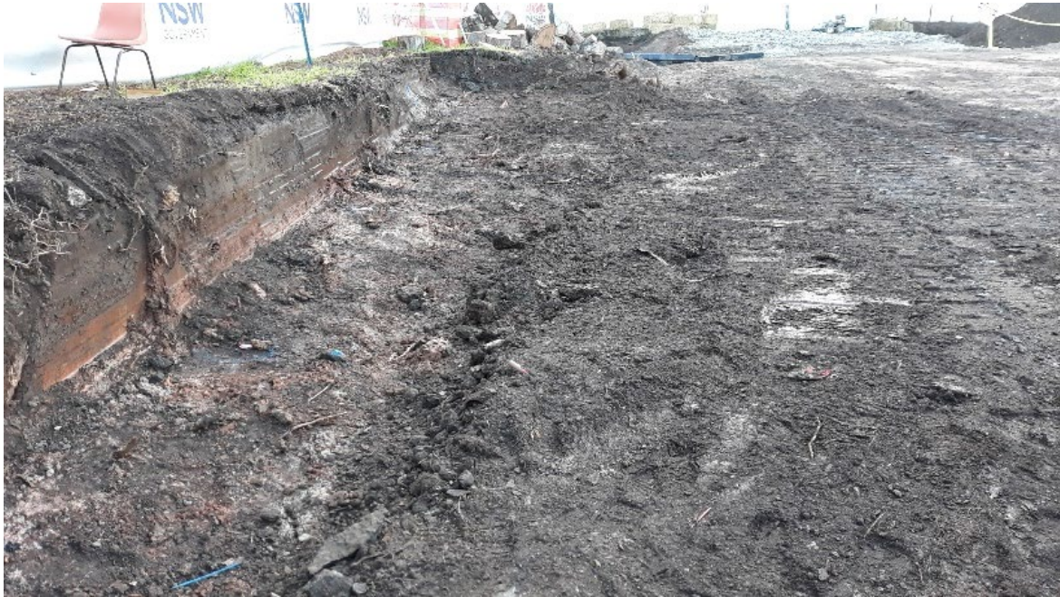
Looking across the Grid 4 and 6 areas at the Penshurst Public School at completion of visual walkover inspection on 1 August 2019
