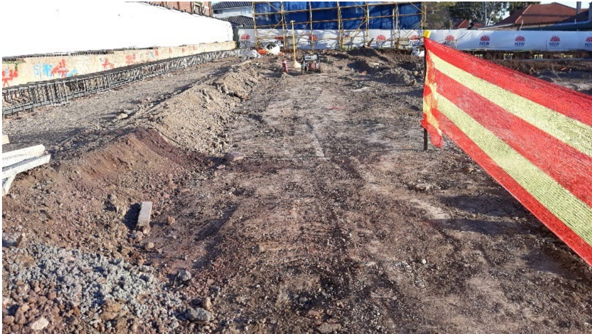
Looking across the Grid 8 area at the Penshurst Public School at completion of visual walkover inspection on 9 August 2019
