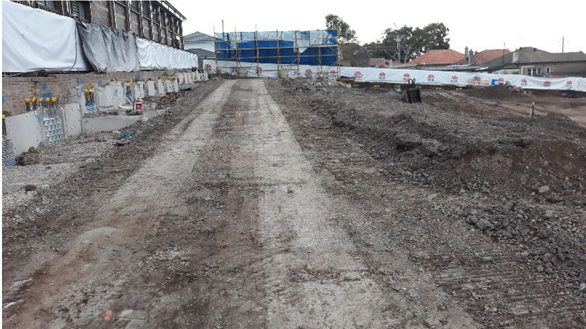
Looking across the Grid 8 area at the Penshurst Public School at completion of visual walkover inspection on 2 August 2019
