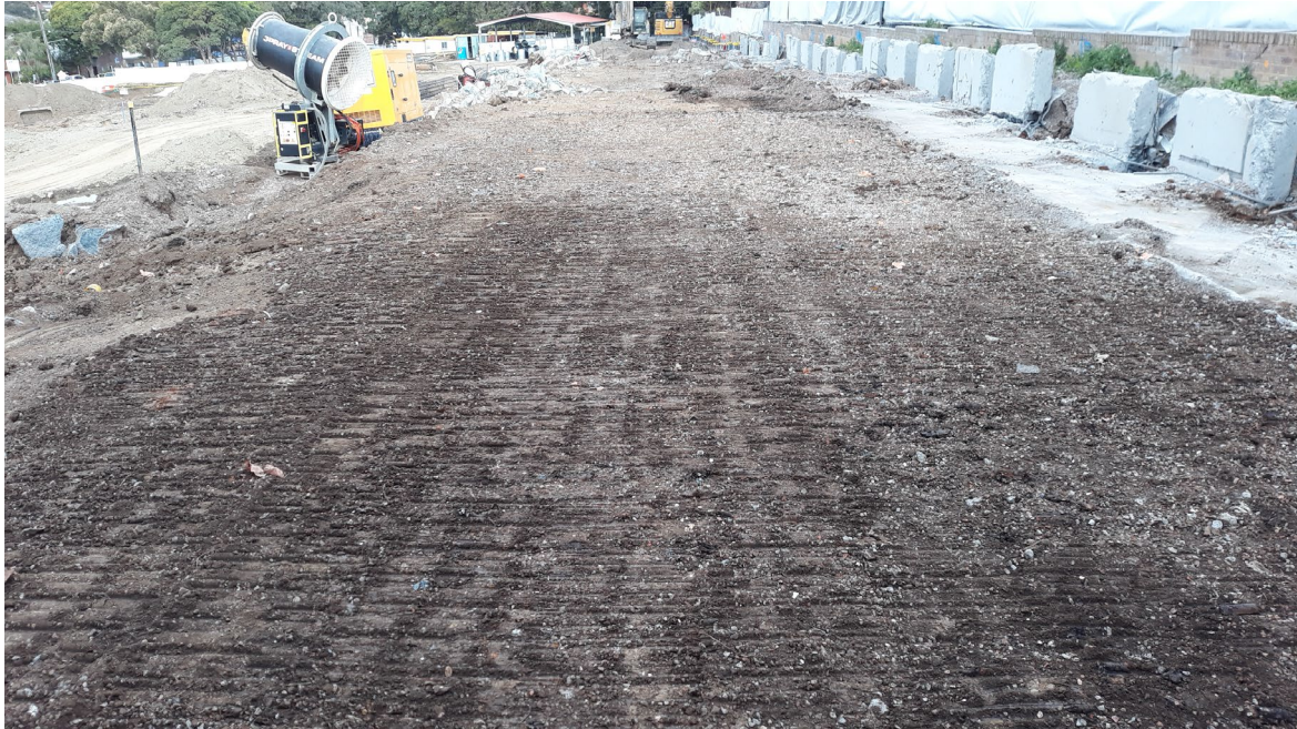
Looking across the Grid 8 area at the Penshurst Public School at completion of visual walkover inspection on 26 July 2019 (afternoon)
