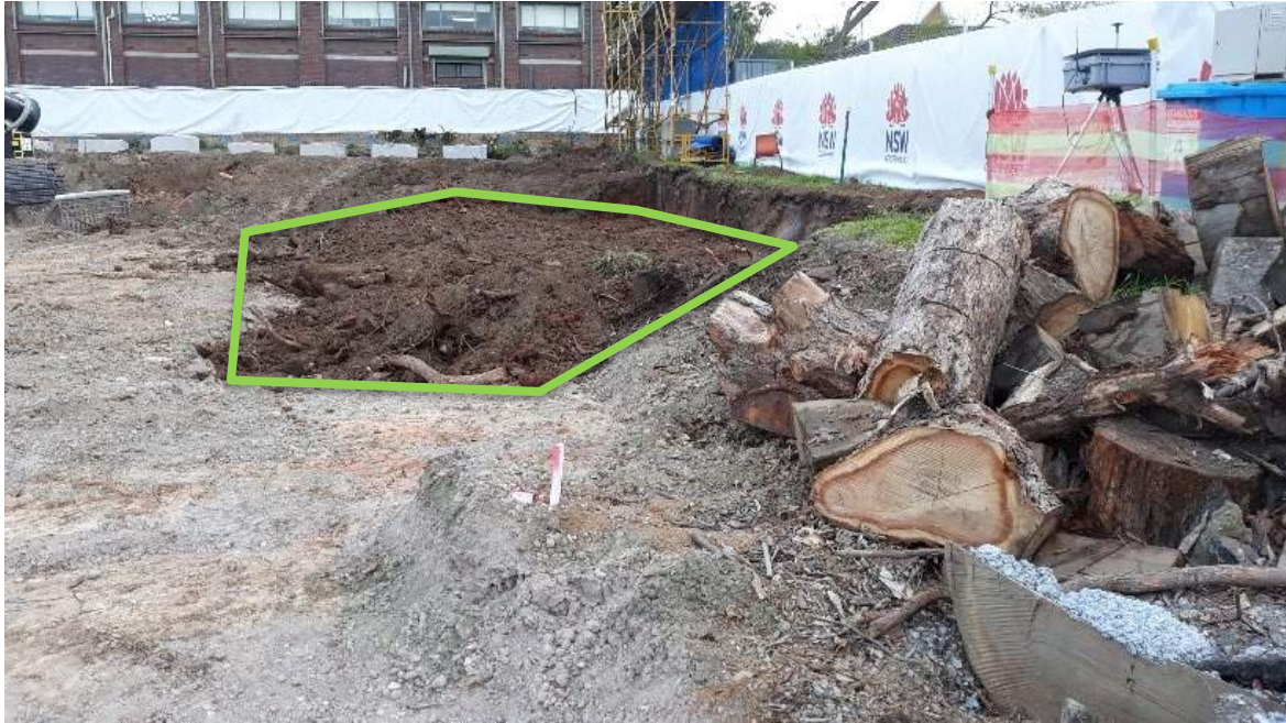
Looking across the Grid 4 and 6 areas at the Penshurst Public School at completion of visual walkover inspection on 29 July 2019 (within green outline)
