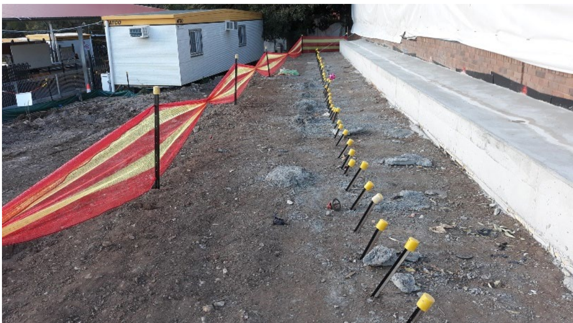
Looking across the Grid 12 area at the Penshurst Public School at completion of visual walkover inspection on 12 August 2019
