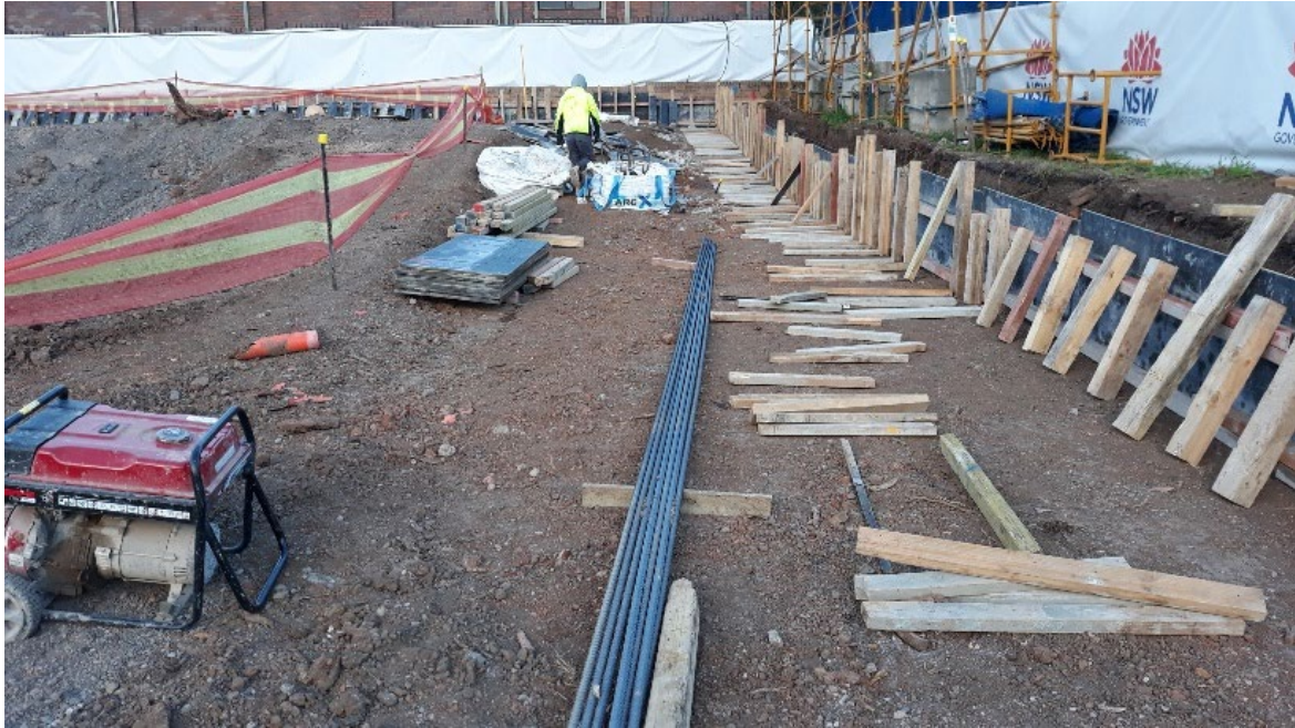
Looking across the Grid 4 and 6 areas at the Penshurst Public School at completion of visual walkover inspection on 12 August 2019
