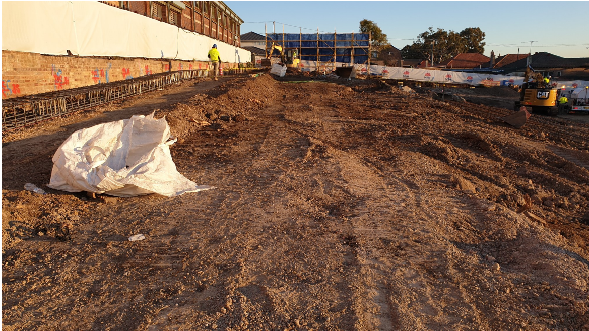
Looking across the Grid 8 area at the Penshurst Public School at completion of visual walkover inspection on 7 August 2019
