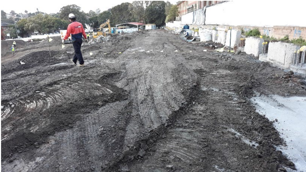
Looking across the Grid 8 area at the Penshurst Public School at completion of visual walkover inspection on 1 August 2019
