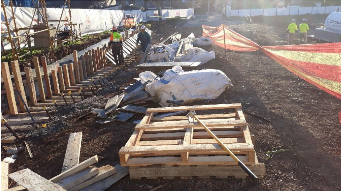
Looking across the Grid 4 and 6 areas at the Penshurst Public School at completion of visual walkover inspection on 14 August 2019
