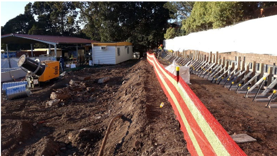
Looking across the Grid 12 area at the Penshurst Public School at completion of visual walkover inspection on 8 August 2019
