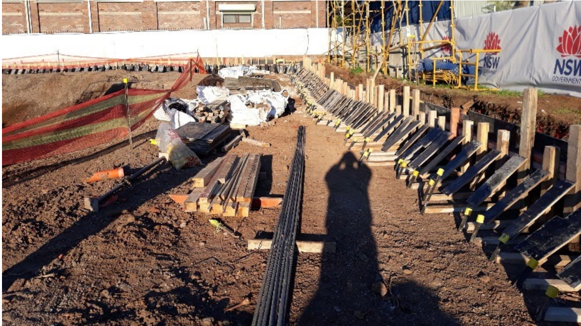
Looking across the Grid 4 and 6 areas at the Penshurst Public School at completion of visual walkover inspection on 13 August 2019
