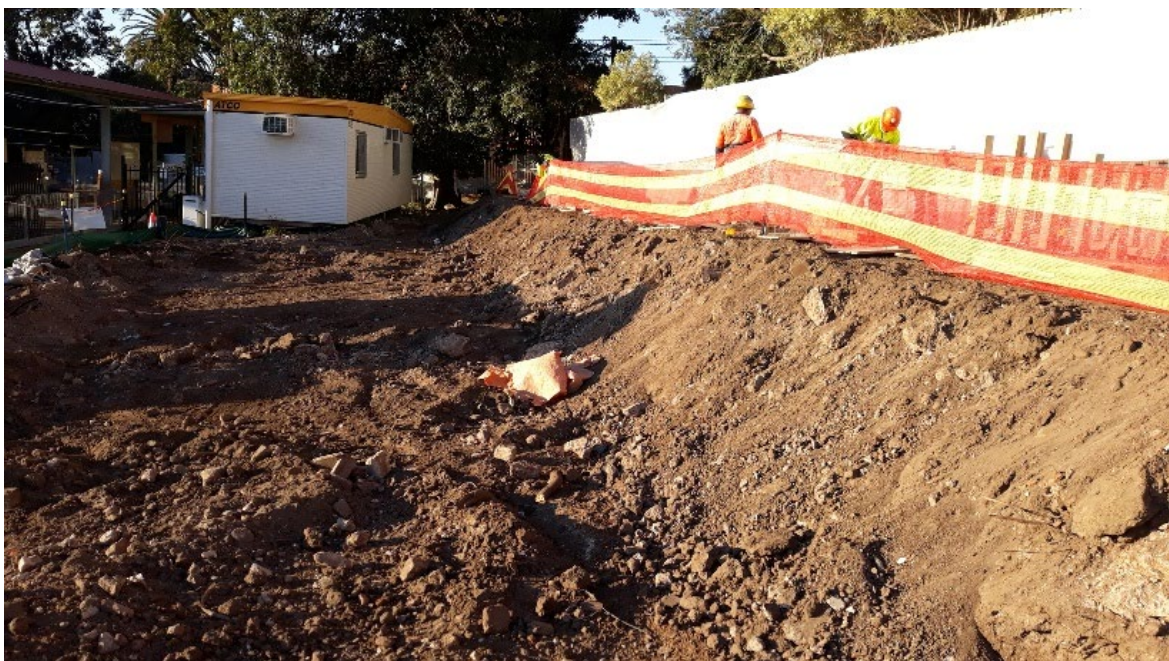
Looking across the Grid 12 area at the Penshurst Public School at completion of visual walkover inspection on 9 August 2019
