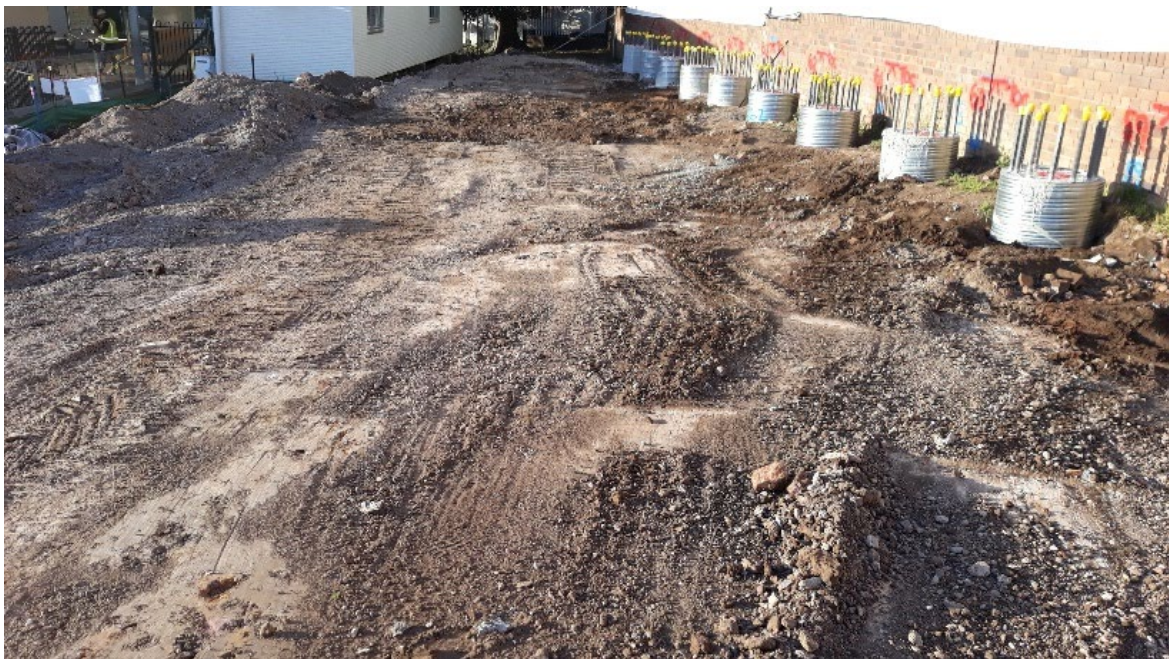
Looking across the Grid 12 area at the Penshurst Public School at completion of visual walkover inspection on 5 August 2019
