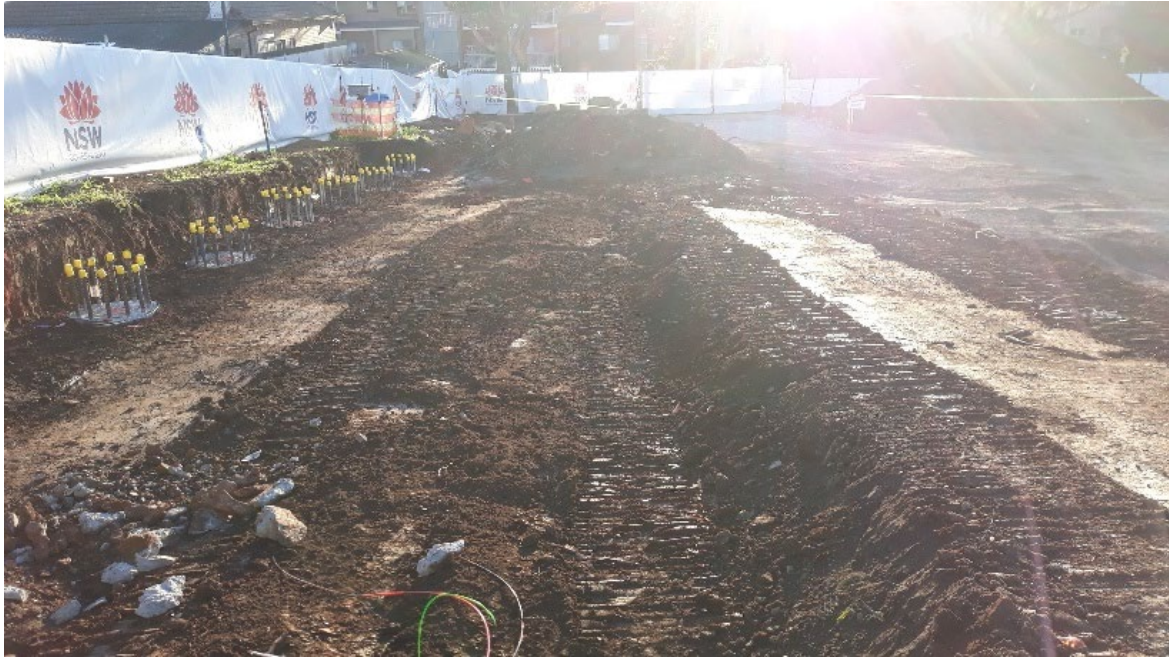
Looking across the Grid 4 and 6 areas at the Penshurst Public School at completion of visual walkover inspection on 8 August 2019
