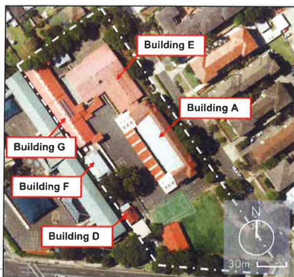
Figure 9 | Identification of existing built form (Source: Applicant's EIS 2018).
