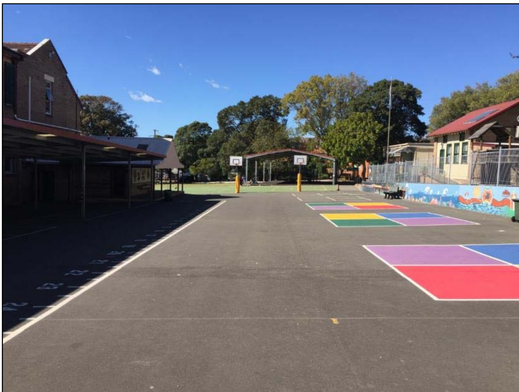
Plate 6: General view across the centre of Penshurst PS looking south east
