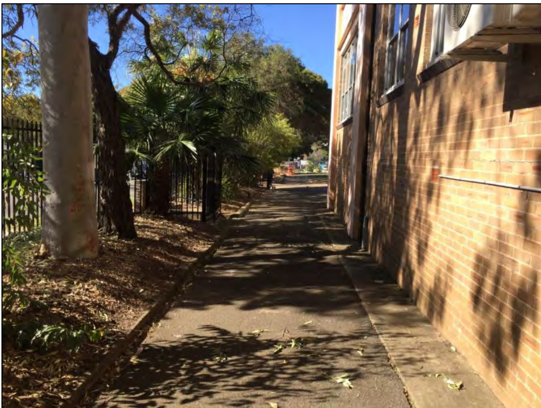
Plate 2: General view looking south east within Penshurst PS.
