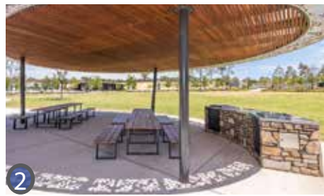
SANDSTONE CLADDING TO BBQ STRUCTURE
