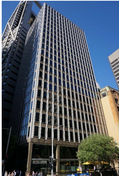
Figure 46 – 1-7 Castlereagh Street, as viewed from Hunter Street
