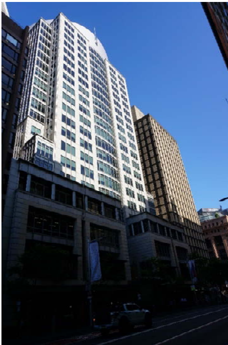
Figure 38 – 60 Castlereagh Street, as viewed from Elizabeth Street
