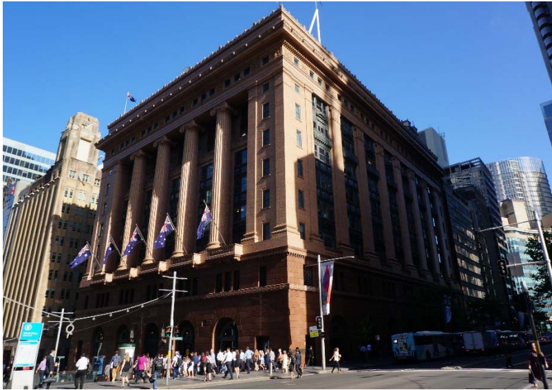
Figure 15 – 50 Martin Place as viewed from Martin Place and Elizabeth Street
