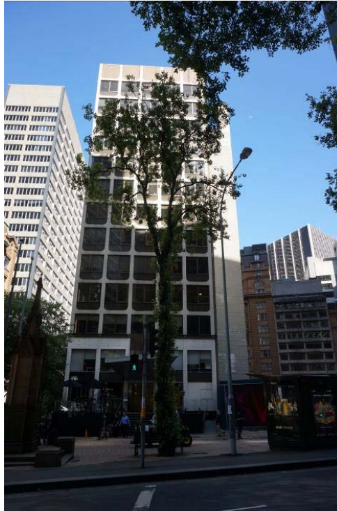
Figure 34 – Richard Johnson Square and 37 Bligh Street, as viewed from Bligh Street
