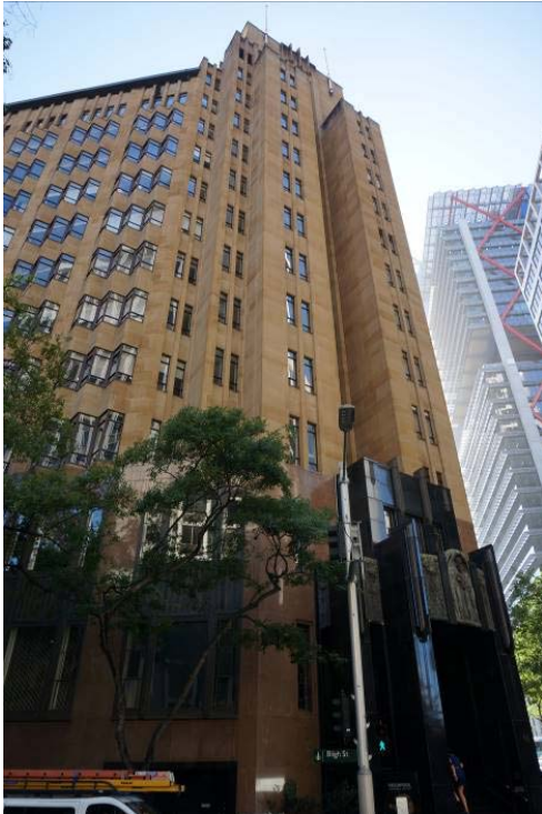
Figure 33 – 60-66 Hunter Street, as viewed from Bligh Street
