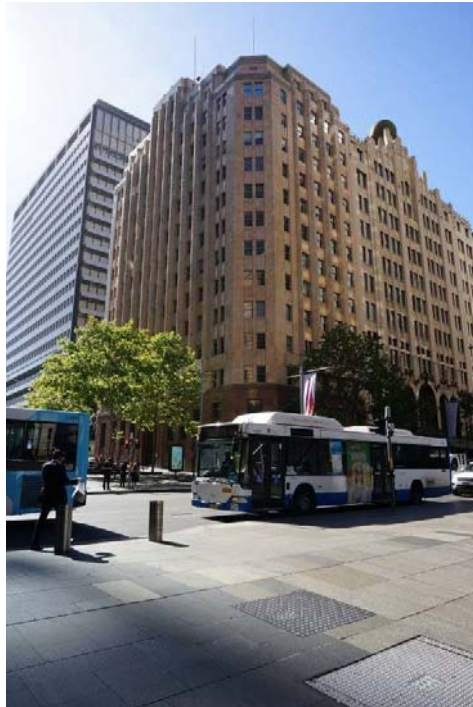
Figure 37 – 53-63 Martin Place, as viewed from Martin Place
