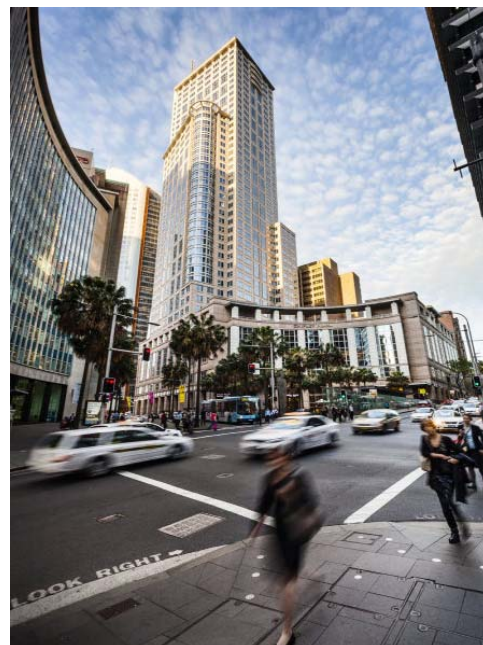
Figure 32 – Chifley Tower, as viewed from the corner of Hunter and Elizabeth Street Source: Colliers International
