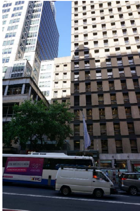
Figure 39 – the South Site building adjoining to 60 Castlereagh Street
