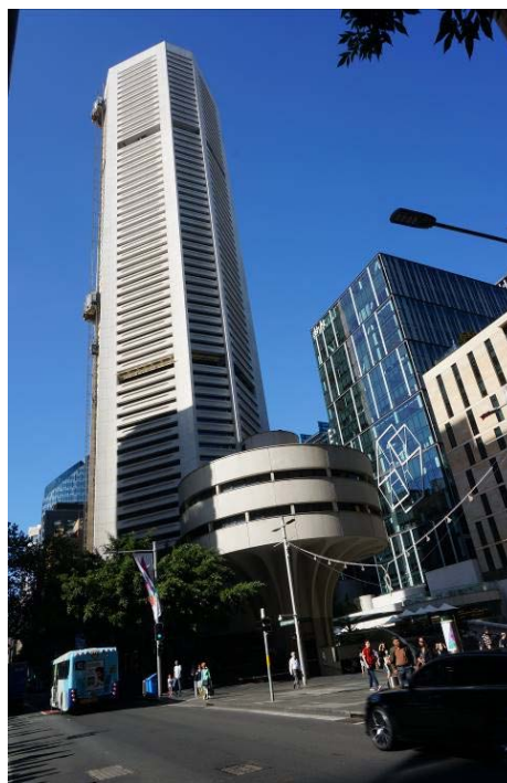
Figure 41 – MLC Centre building as viewed from Martin Place
