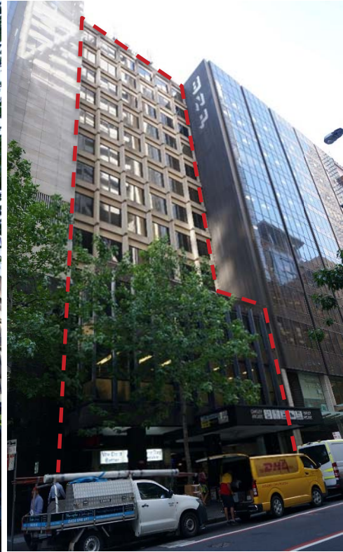
Figure 21 – 5 Elizabeth Street (highlighted in red), as viewed from Castlereagh Street
