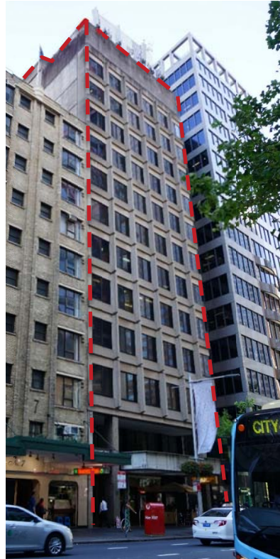
Figure 20 – 5 Elizabeth Street (highlighted in red), as viewed from Elizabeth Street
