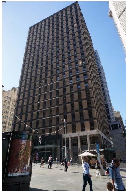
Figure 26 – 39-49 Martin Place, as viewed from Martin Place Street
