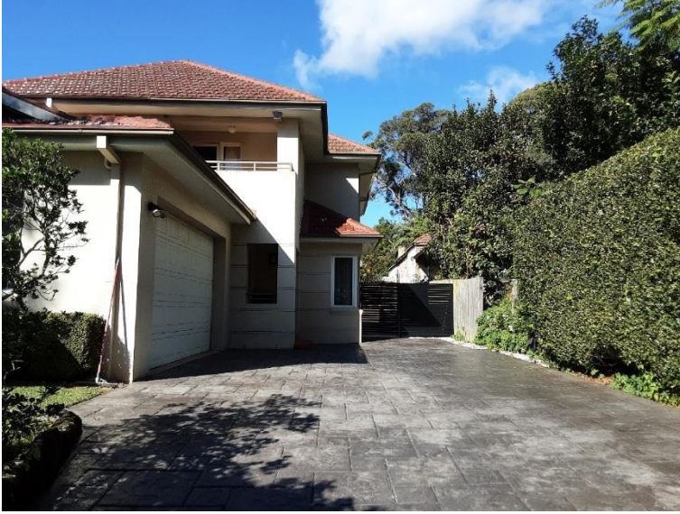
Photo 25 The paths and driveway [17] of new dwelling in number 21 [15], facing south
