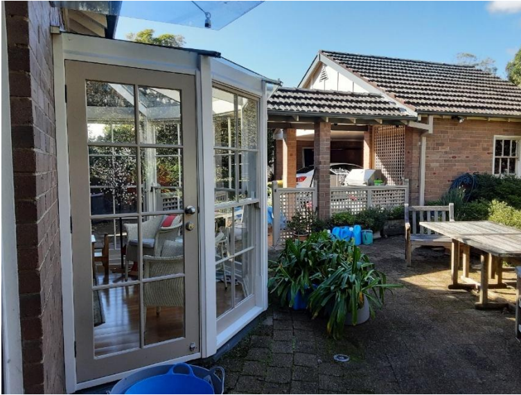
Photo 30 The rear structure [20] of the dwelling in number 23 and formal garden paving [28], also showing previous locations of the two rear outbuildings [7] and [8], facing east
