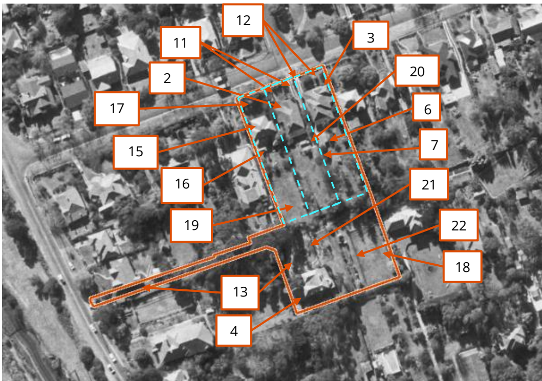
Photo 16 1970 aerial with the study area outlined in red showing demolished structures [5] and new structures [21] [22] (Source: NSW Spatial Services 2025)
