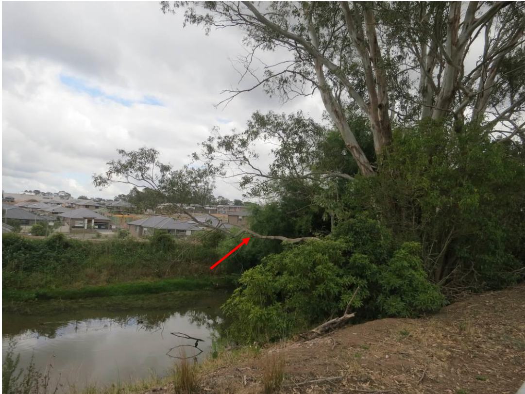
Image 3 – Photo taken from south-west, showing lateral branch over dam that will require removal
