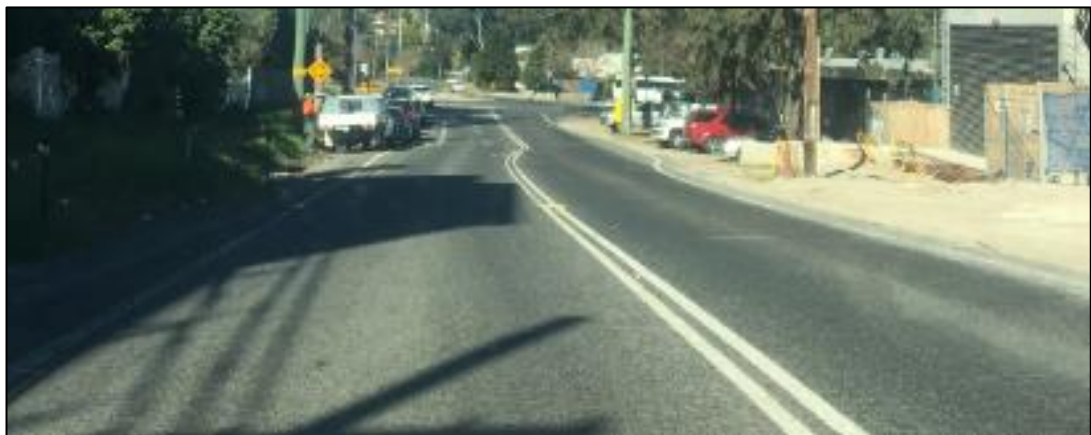
Figure 2-5 – Hezlett Road at Samantha Riley Drive (facing south)
