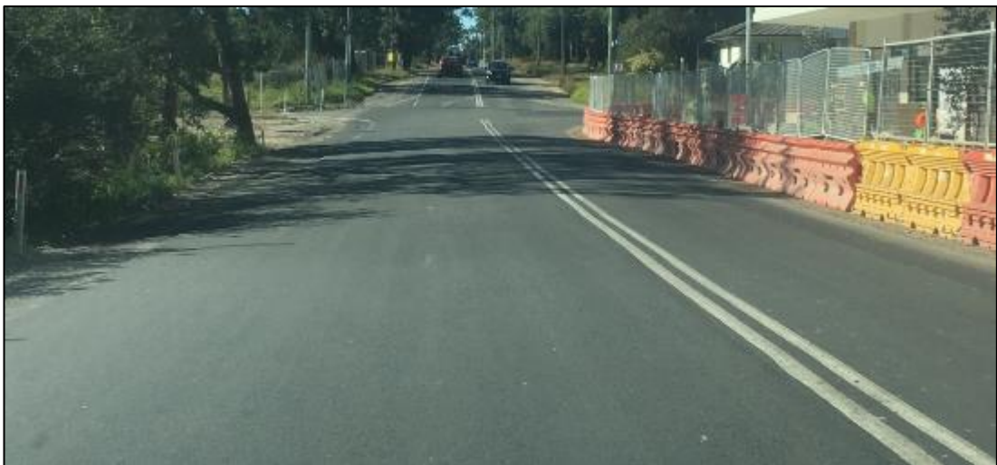
Figure 2-9 – Withers Road at Hezlett Road (facing east)
