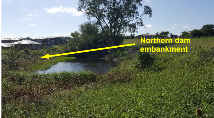
Photograph 2 – Dam 1: View of Dam from western side
