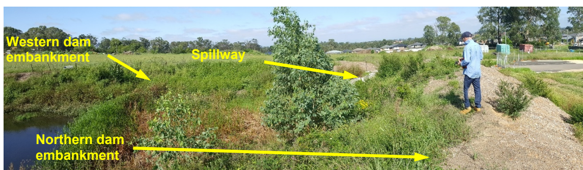
Photograph 1 – Dam 1: View of dam embankment and spillway from eastern side
