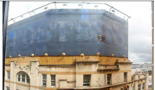
Existing situation – view from adjoining hotel
