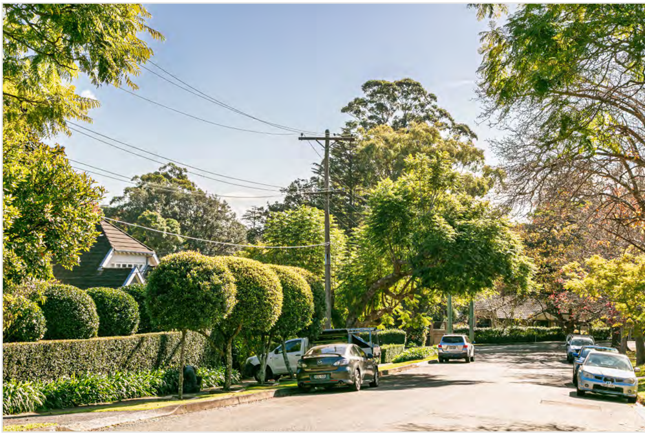
Existing site photo - Waimea Road pavement
