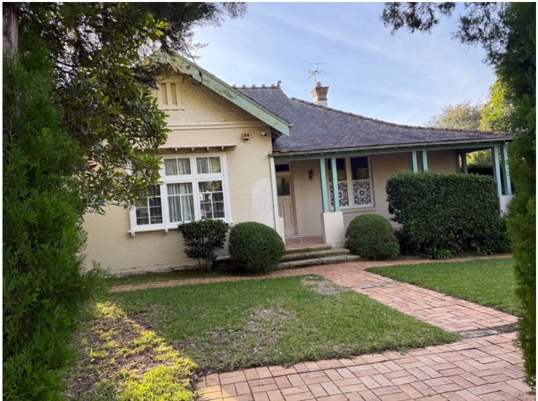
Figure 3: No 16 Middle Harbour Road as viewed from the street.
