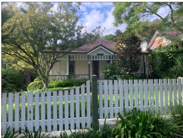
Figure 20: No. 9 Lindfield Avenue from Lindfield Avenue.
