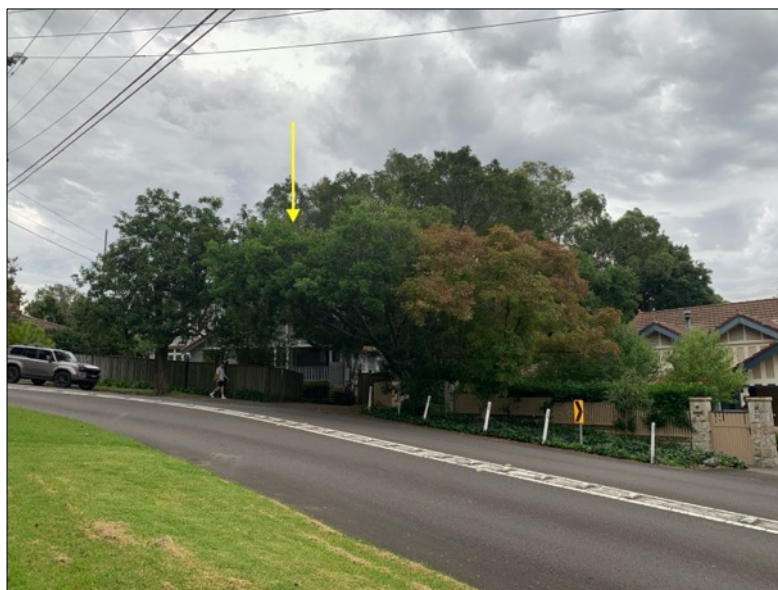
Figure 35: Second view out of the Clanville Conservation Area towards the subject site, marked by the arrow, from Strickland Avenue. The proposed building may be visible in this view corridor behind the No. 27 Strickland Avenue.
