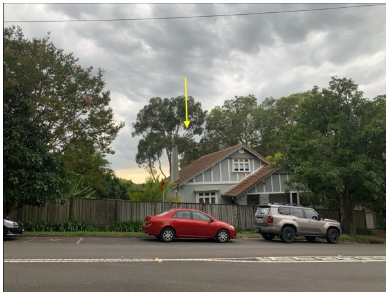
Figure 34: View out of the Clanville Conservation Area towards the subject site, marked by the arrow, from Strickland Avenue. The proposed building may be visible in this view corridor, behind the No. 27 Strickland Avenue.
