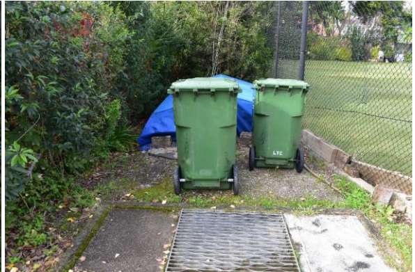
Figure 32: view southeast of subsurface water works along the northern boundary of the walkway
