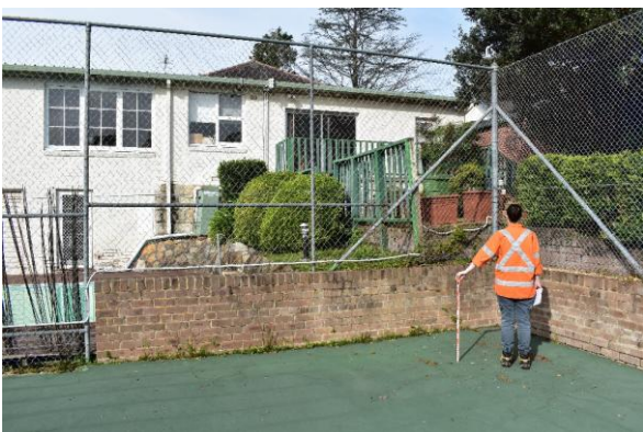
Figure 19: terracing levels indicating distinct cuts into the landscape and retaining walls to separate the inground pool and tennis court.
