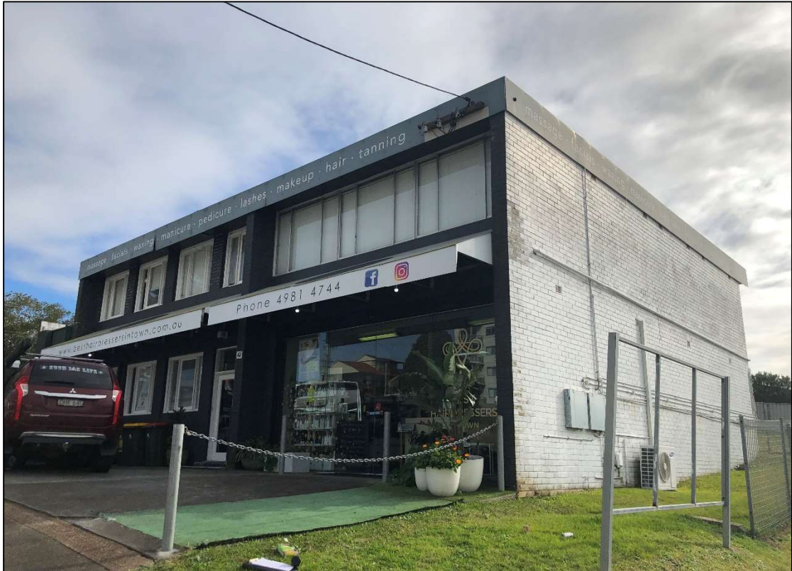
Photo 19: Commercial building, Lot B, looking north west
