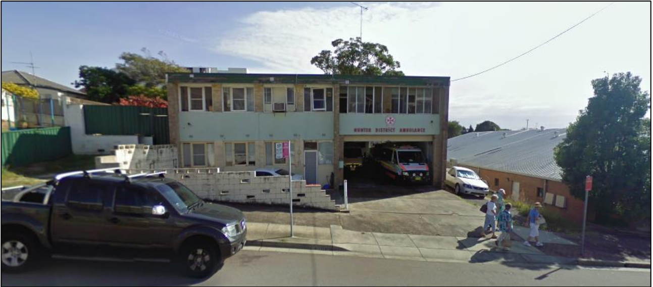
Figure 4: 2010 street level photography, Lot B DP 417172 (photograph sourced from Google Street View).
