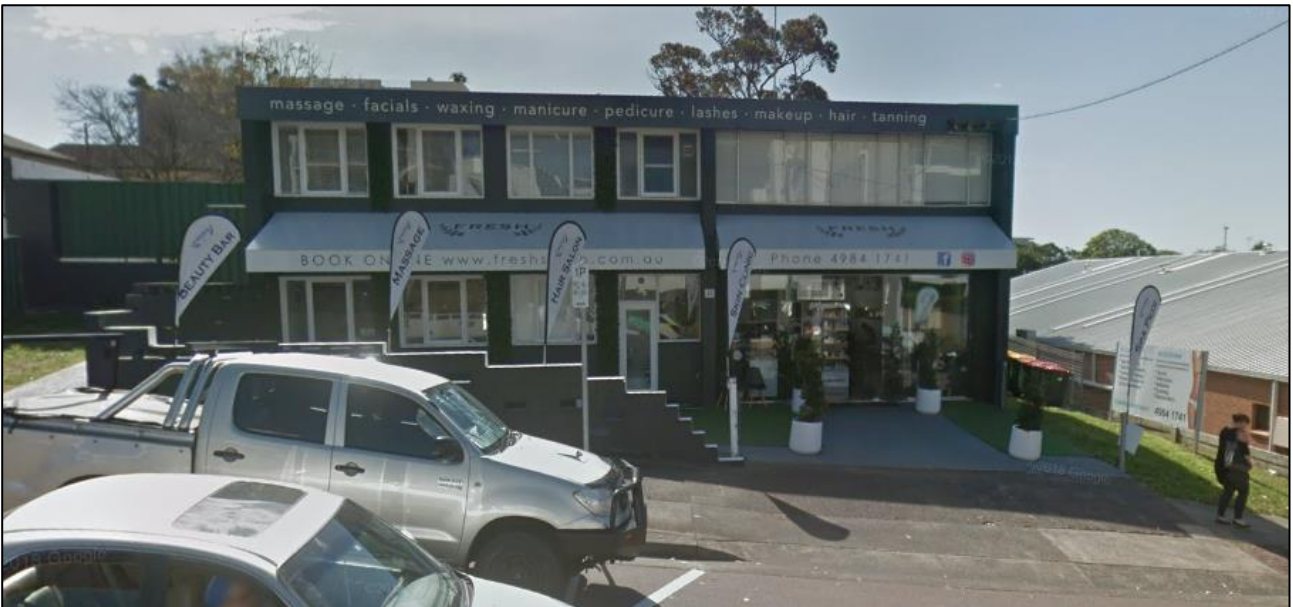
Figure 5: 2017 street level photography, Lot B DP 417172 (photograph sourced from Google Street View).
