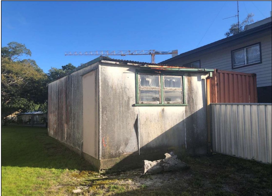
Photo 9: Garage, Lot 15, looking north west
