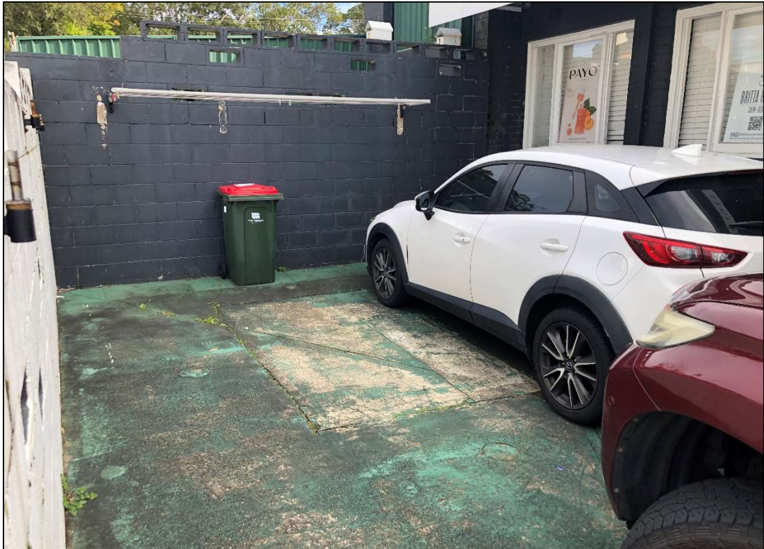
Photo 20: Concreted area, Lot B, looking west
