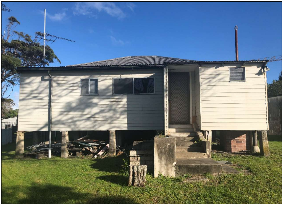
Photo 6: Residential dwelling, Lot 15,, looking west
