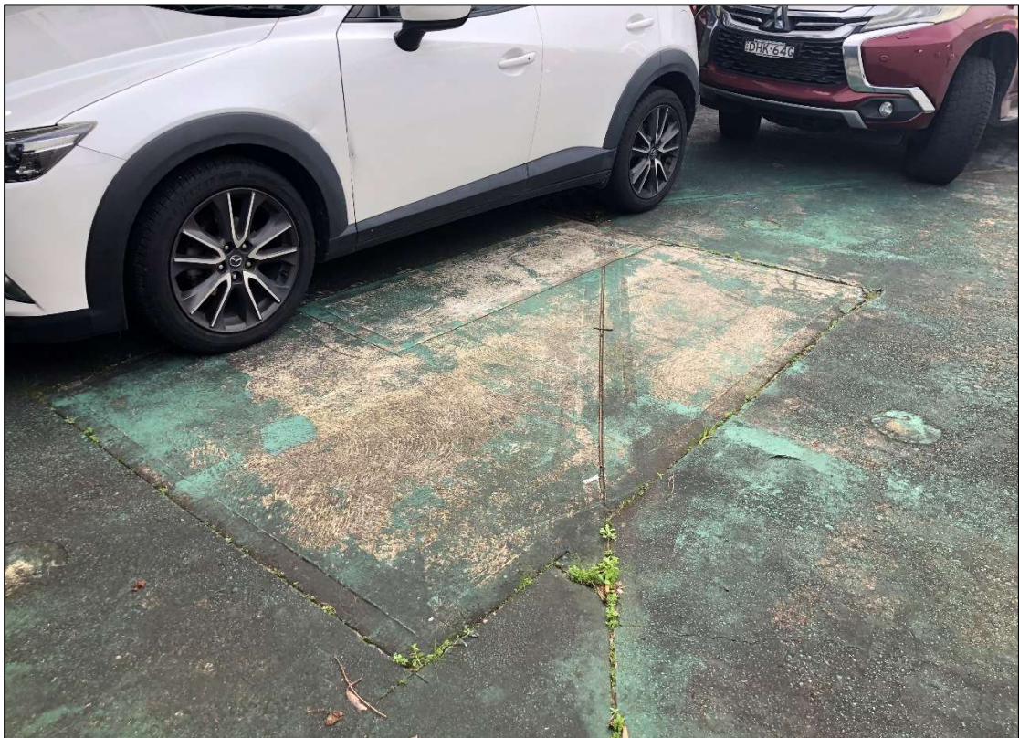
Photo 21: Concreted area, Lot B, looking north east
