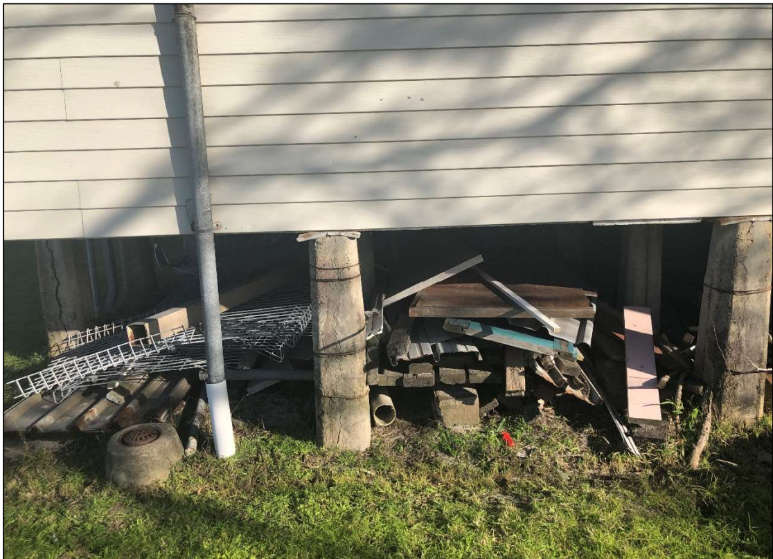
Photo 7: Stockpiles of materials, subfloor of residential dwelling (Lot 15), looking west
