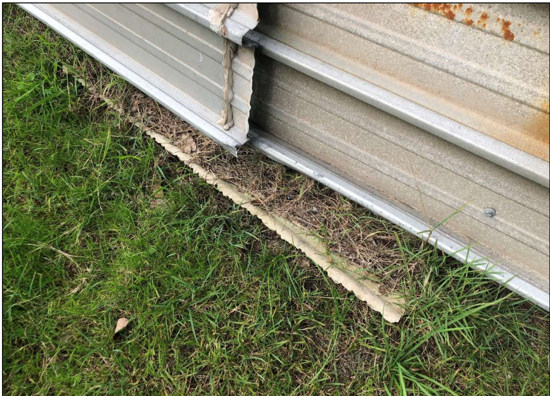
Photo 14: Fibro sheeting, Lot 15, looking east
