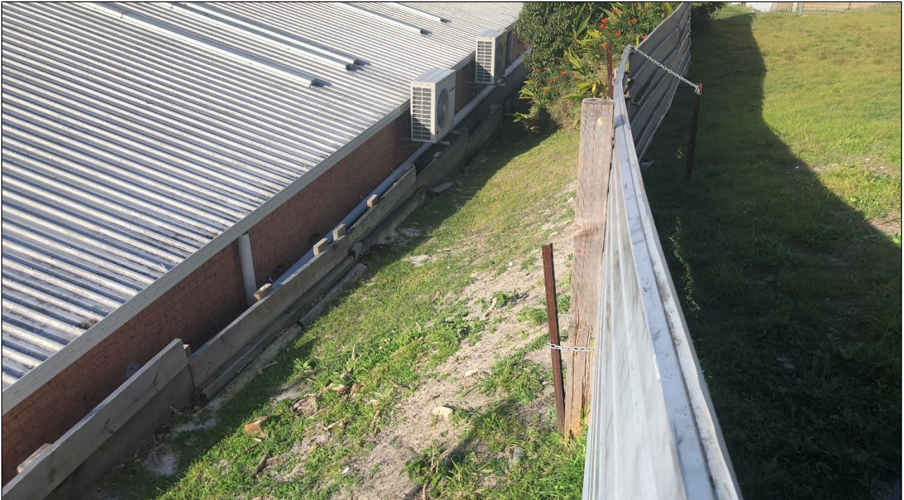
Figure 6: Looking approximately south along the eastern site boundary. Note existing timber retaining wall, estimated to be up to 3 m in height for adjacent commercial property.
