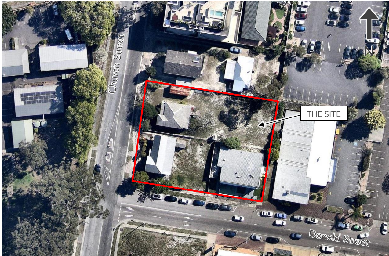
Figure 2 – Pre-Developed Site Condition (Nearmap image dated – 09.09.2018)
