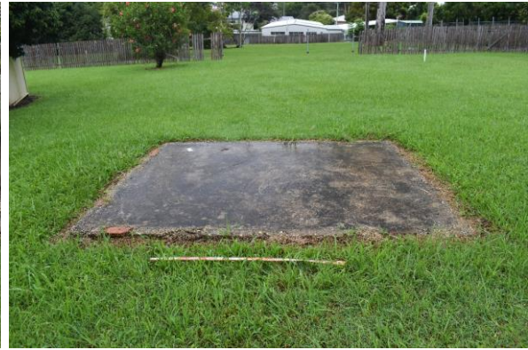
Figure 31: View of cement foundation with brick lining
