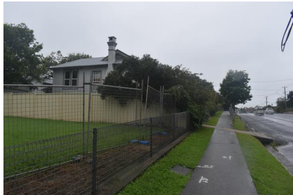
Figure 45: View southeast from study area entrance to northwest face of extant courthouse boundary
