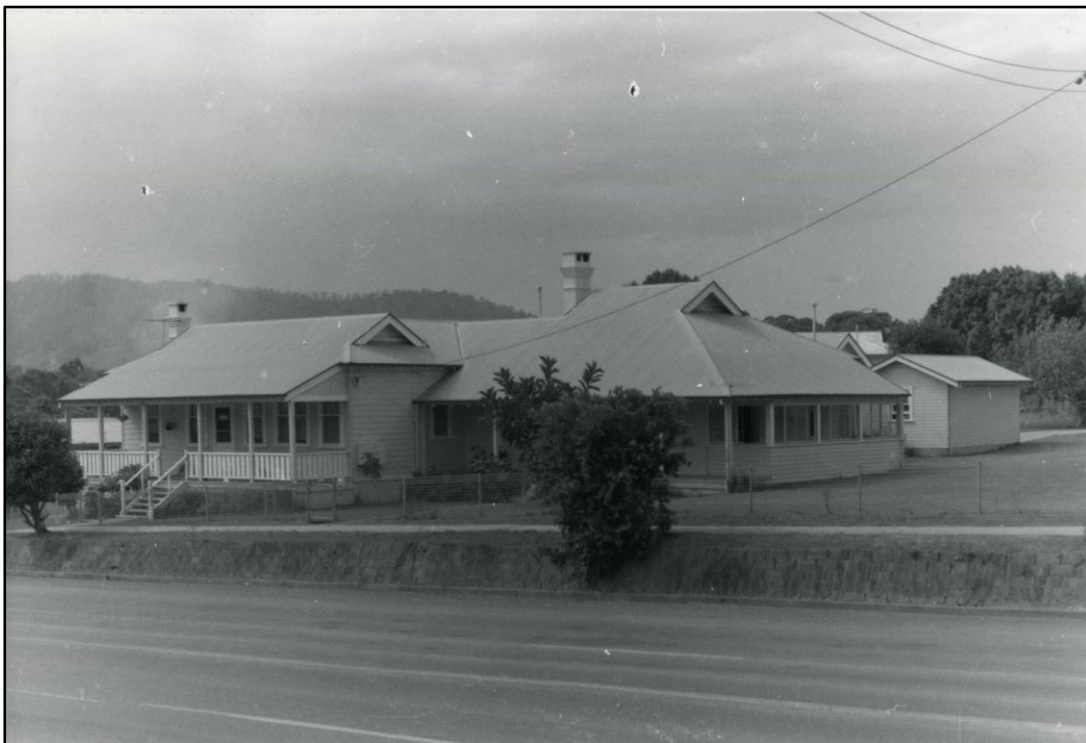
Figure 7: Police station and Courthouse, February 1982 (Source: Coffs Collection accession number. M2022.70.2)
