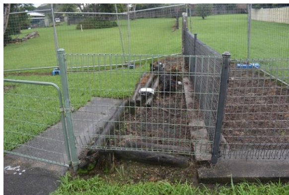
Figure 37: view of disturbance at front of site abutting Harbour Drive road
