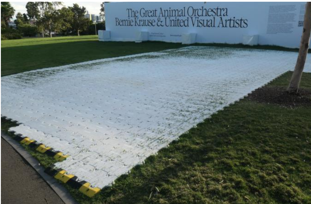
Figure 3.2 – Example of acceptable Tree Protection Area ground protection (Photo: Arterra)
