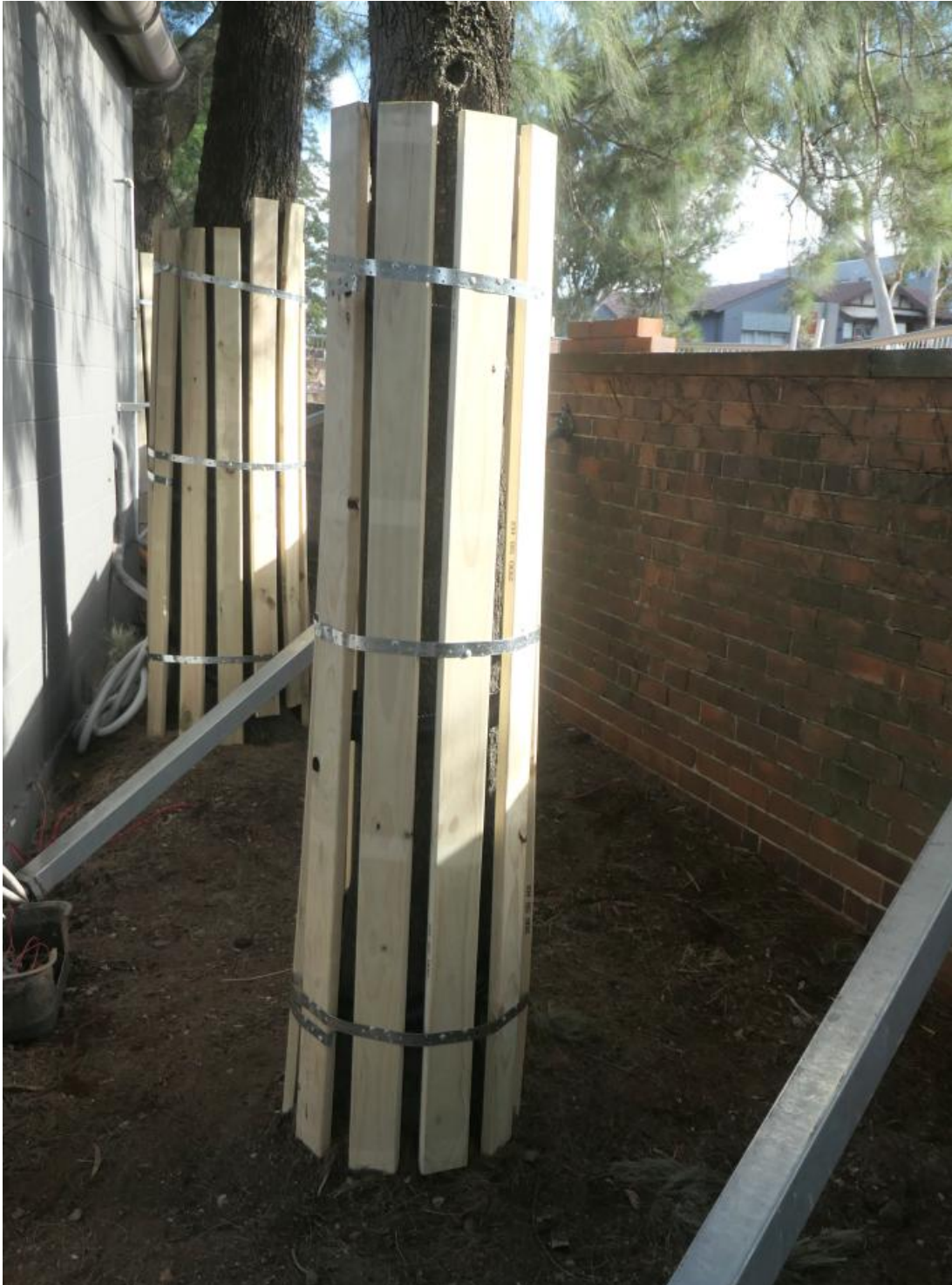
Figure 3.3– Example of acceptable Trunk Protection batten installation. (Photo: Artera)
