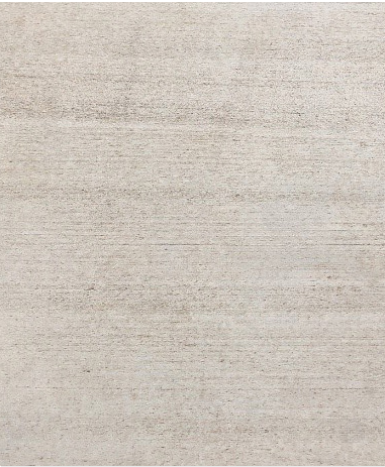
Concrete Paving Broom Finish
