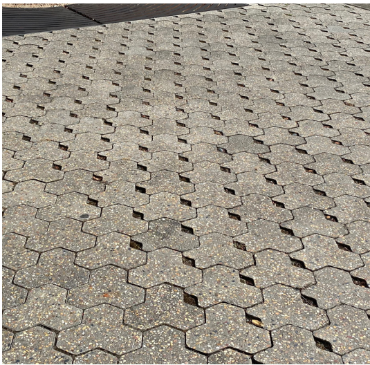
Permeable paving
