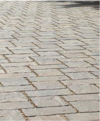
Permeable Unit Pavers
