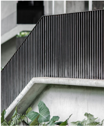
METAL PALISADE BALUSTRADE
