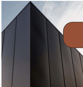
METAL WALL CLADDING TO BALCONY INTERIORS; LYSAGHT 'EXPRESSION' INTERLOCKING WALL SYSTEM OR EQUIV. COLOUR SIMILAR TO COLORBOND ARIES OR EQUIVALENT
