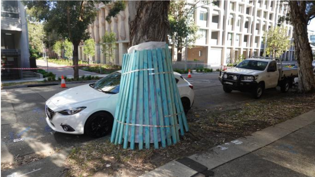
Figure 19 – Example of acceptable Trunk Protection batten installation. (Photo: Arterra)
