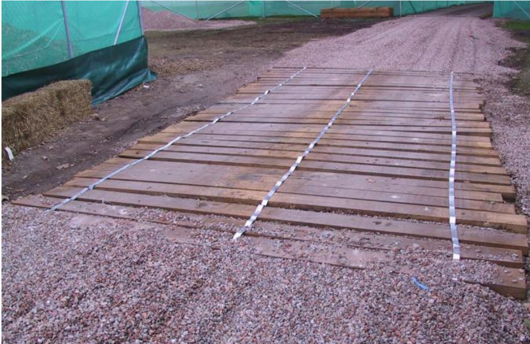
Figure 17 – Example of acceptable Tree Protection Area ground protection (Photo: Arterra)
