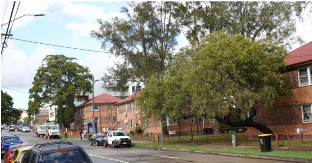
Figure 2 – View of the site from Burwood Road showing the two-storey red brick walk-up residential flat buildings with trees of varying retention value fronting the street. (Photo: Arterra 24 April 2025)
