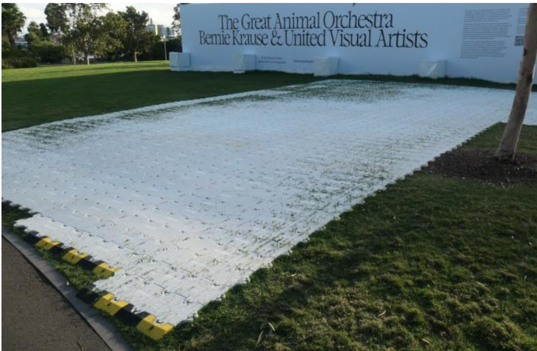
Figure 18 – Example of acceptable Tree Protection Area ground protection (Photo: Arterra)
