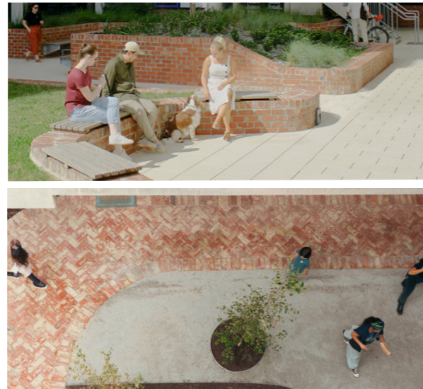
Reuse on-site mixed colour bricks for paving
