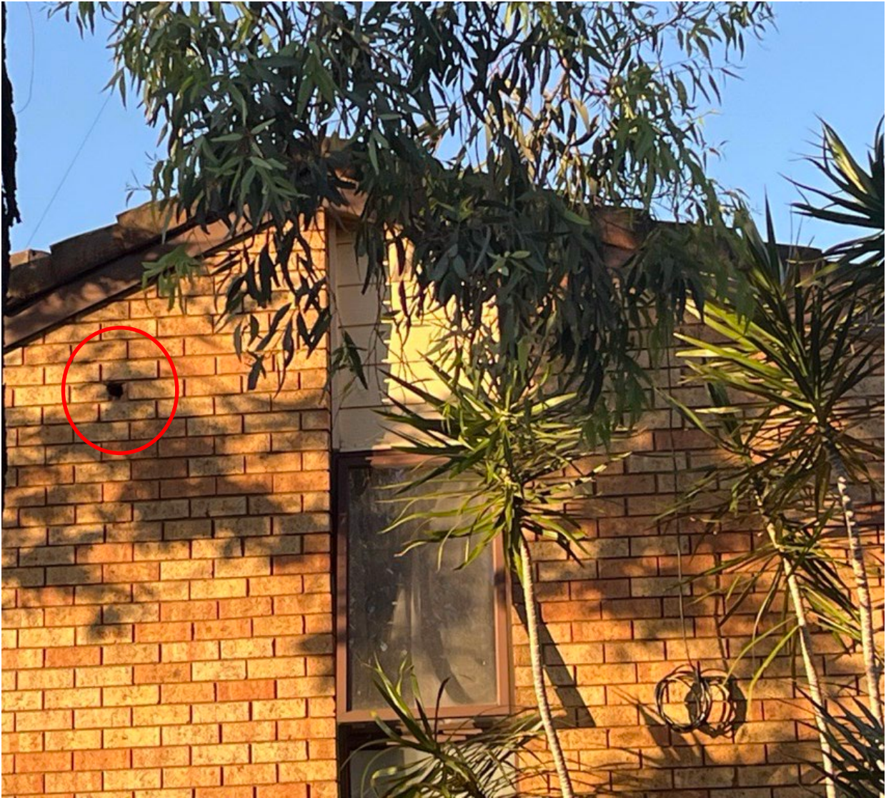
Figure 13: Example of potential entry/exit point into exterior brick wall cavity observed on one building, which may provide access to roosting habitat for microbats.
