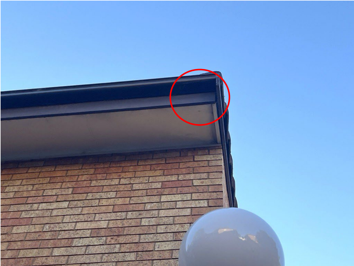
Figure 14: Potential entry/exit point into roof cavities observed on another building, which may provide access to roosting habitat for microbats.
