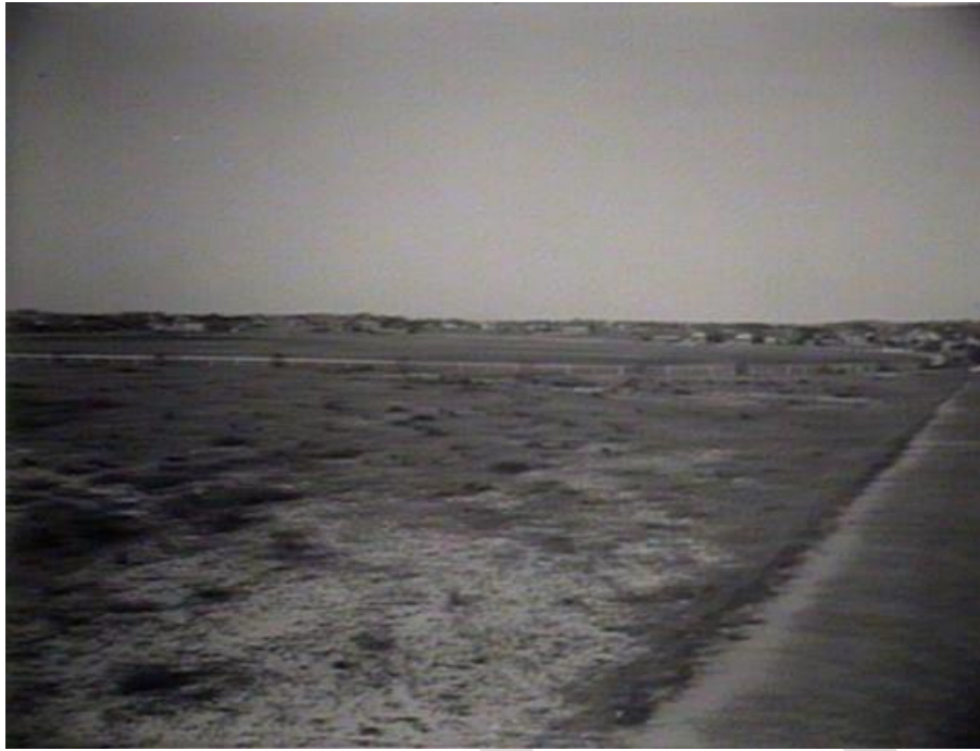
Figure 3-20: Jellicoe Park levelling, grassing & tar banking, showing the appearance of the area's remnant sand dunes by this date. (April 1934). Source: State Library of NSW (Record Identifier: 9yMd8jA9).
