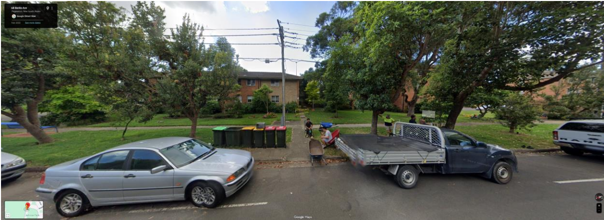
Figure 3-33 68-70 Banks Avenue section of study area as viewed from Banks Avenue, looking east. Source Google Streetview, accessed September 2025
