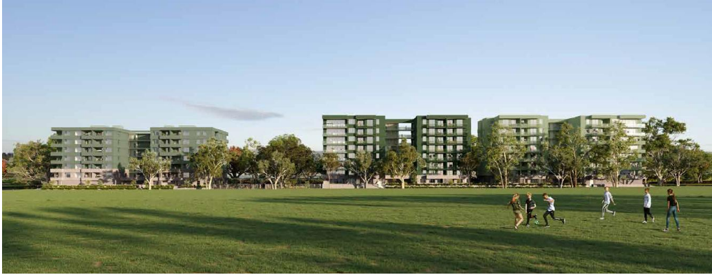
Figure 7.3: Visualisations showing view looking west from Jellicoe Park. Source: Architectural Design Report BVN Architects October 2025
