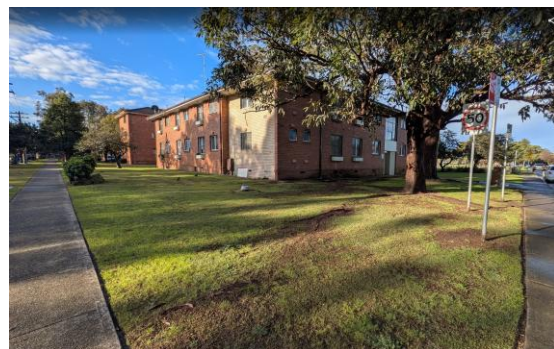
Figure 3.3. Study area as viewed from Banks Avenue, looking north. Source: Curio Projects, August 2025.
