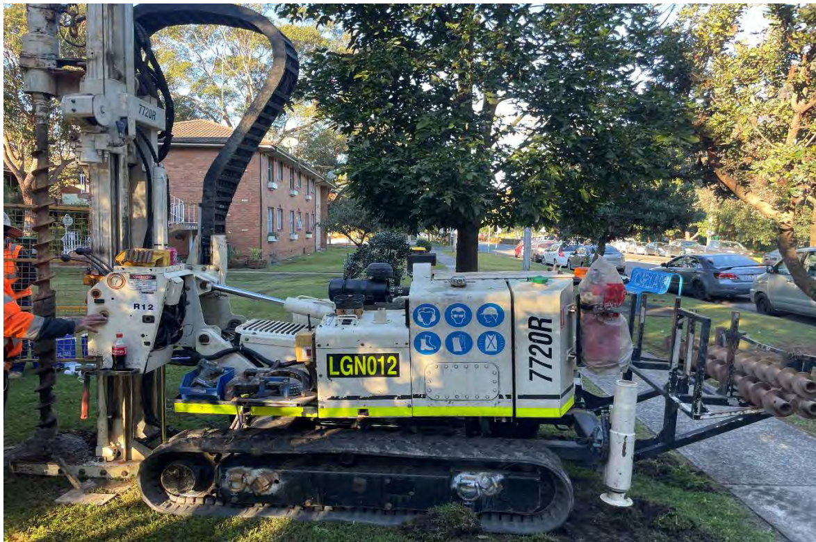
Photo 3 - Typical Setup of a Geoprobe 7720R Track-Mounted Drill Rig
