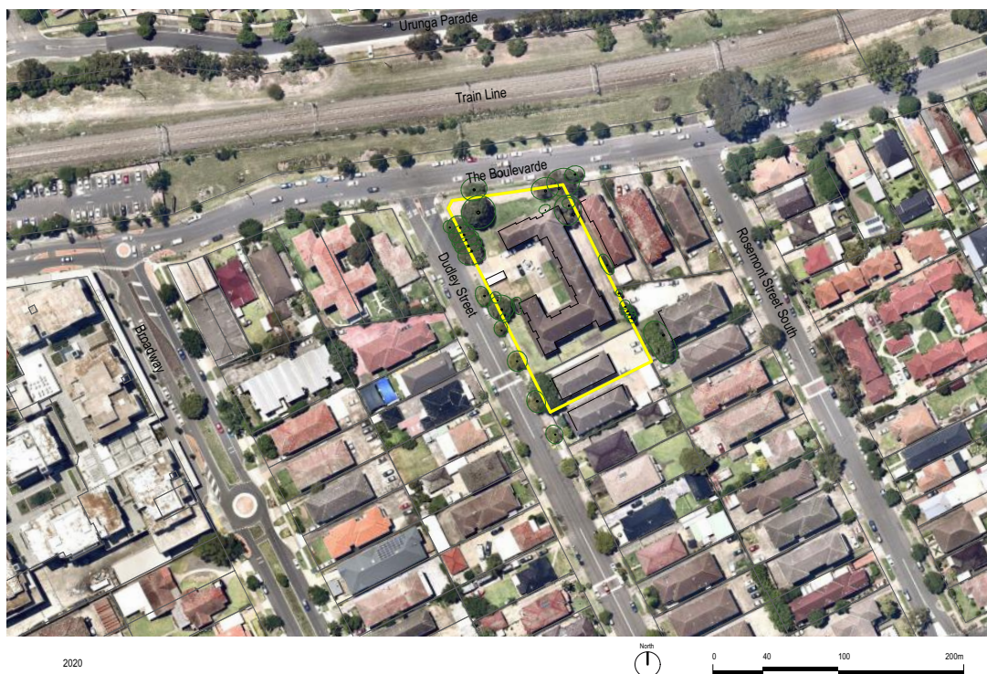
Figure 2.8– Aerial image of the site in 2020 illustrating the site. The site and its trees appearing largely as it occurs today. (Source: Arterra / NearMap)
