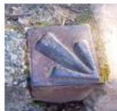
Alignment Pin references road alignment
