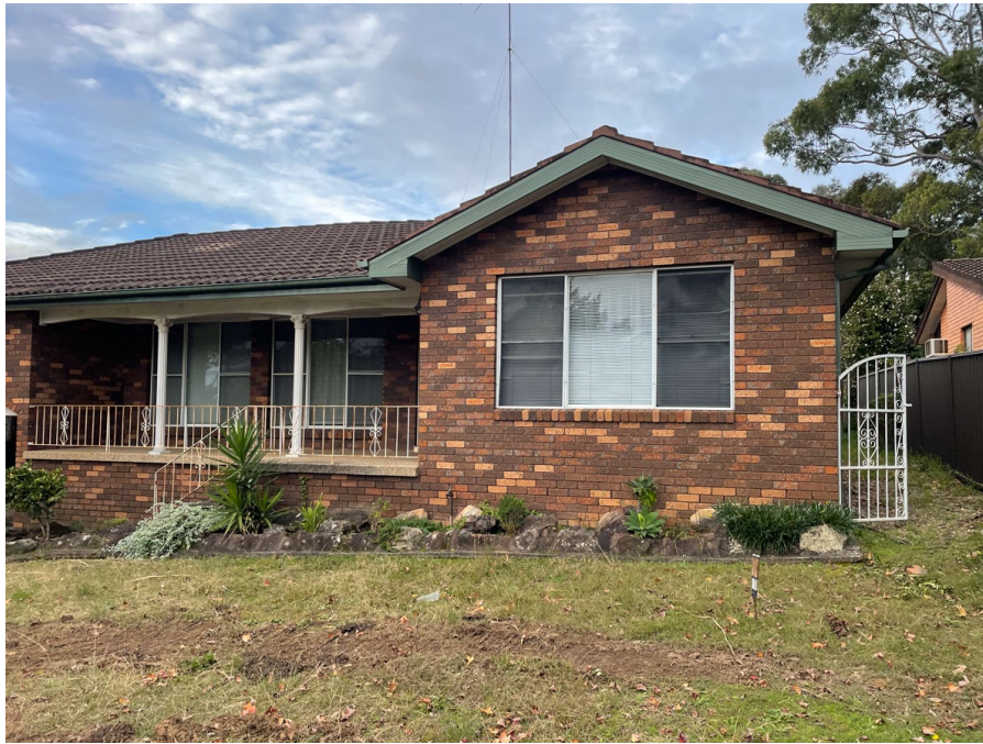
AS11: 6 Middleton Avenue, front veranda ceiling
