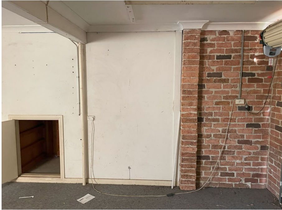
AS7: 4 Middleton Avenue, ground floor bathroom walls
