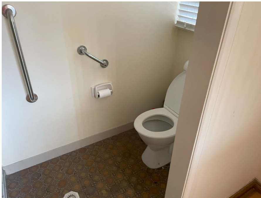
AS6: 4 Middleton Avenue, ground floor bathroom walls
