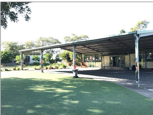
Picture 5 – Looking East: Existing COLA Source: Urbis
