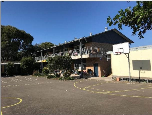
Picture 3 – Looking South-East: Existing Block M Source: Urbis
