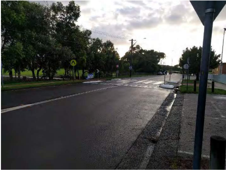
View looking east on Abbott Road showing Raised Zebra Crossing
