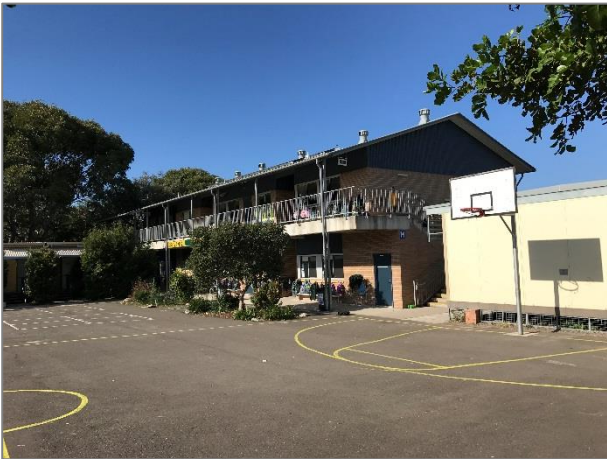
Picture 3 – Looking South-East: Existing Block M
