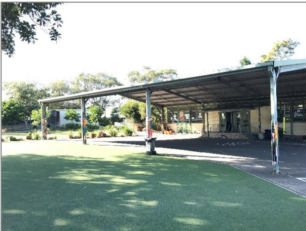
Picture 5 – Looking East: Existing covered outdoor learning area
