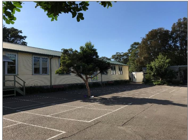
Picture 4 – Looking North-East: Existing Classrooms
