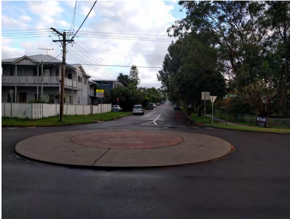
View of the Abbott Road and Playfair Road Roundabout Intersection
