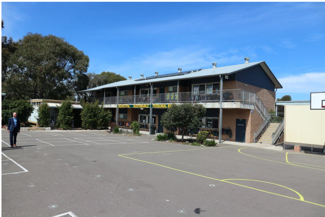
Block M, flanked by demountables. The most recent permanent structures on site are compliant with current Building Codes.
