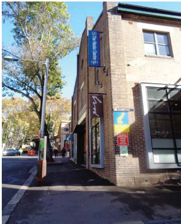
Site Photo 4 - Heritage building, looking toward the north-west (up-slope), May 2017.
