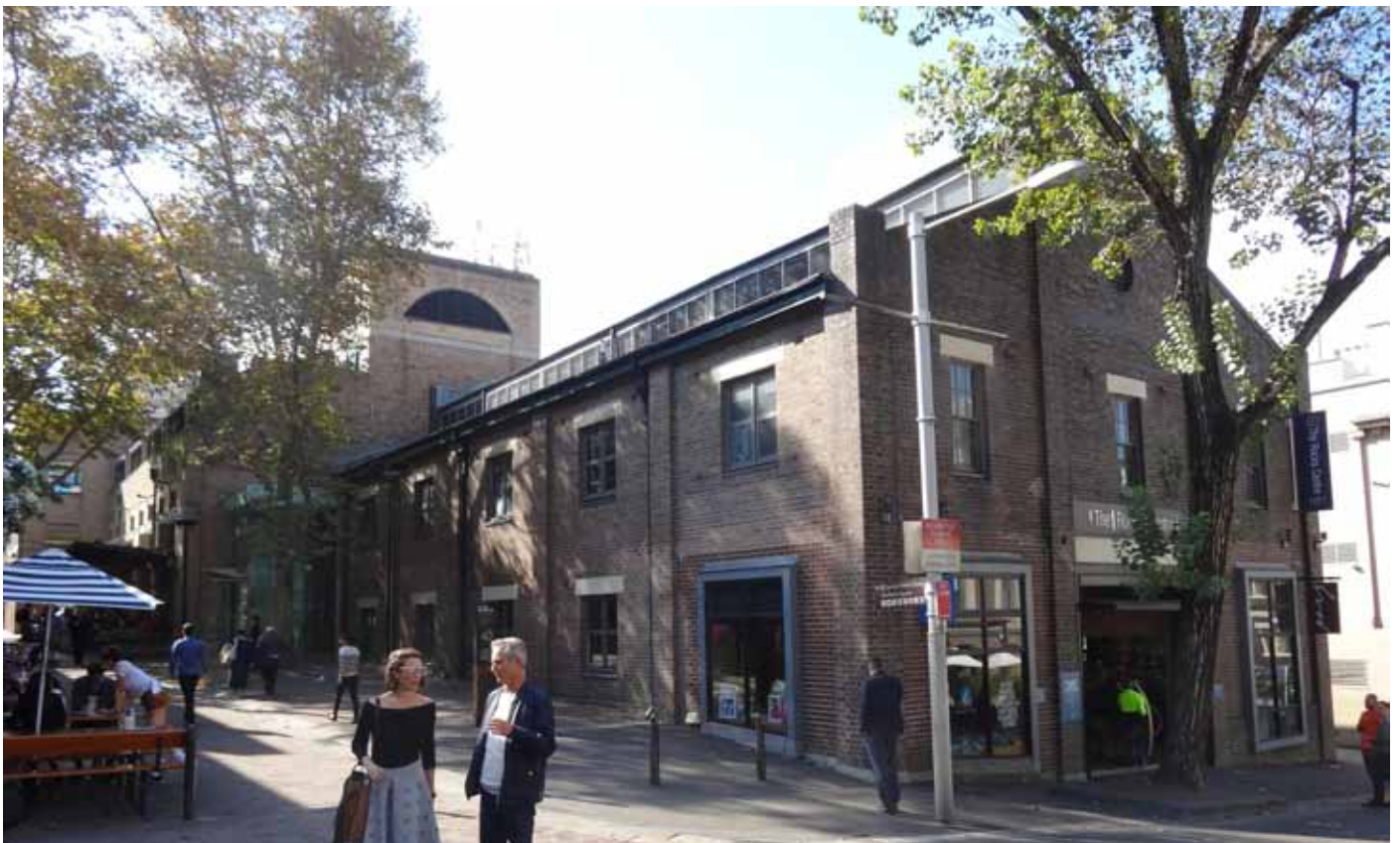
Figure 2.16 The building today with its adaptive use.
