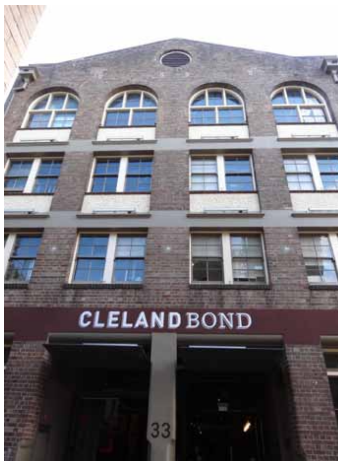
Figure 2.12 The Cleland Bond building is a former warehouse and one of the first buildings re-adapted for new use as an office space.
