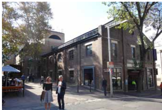
Figure 2.1 View of The Penrhyn House showing the existing glazed entrance in the background.
