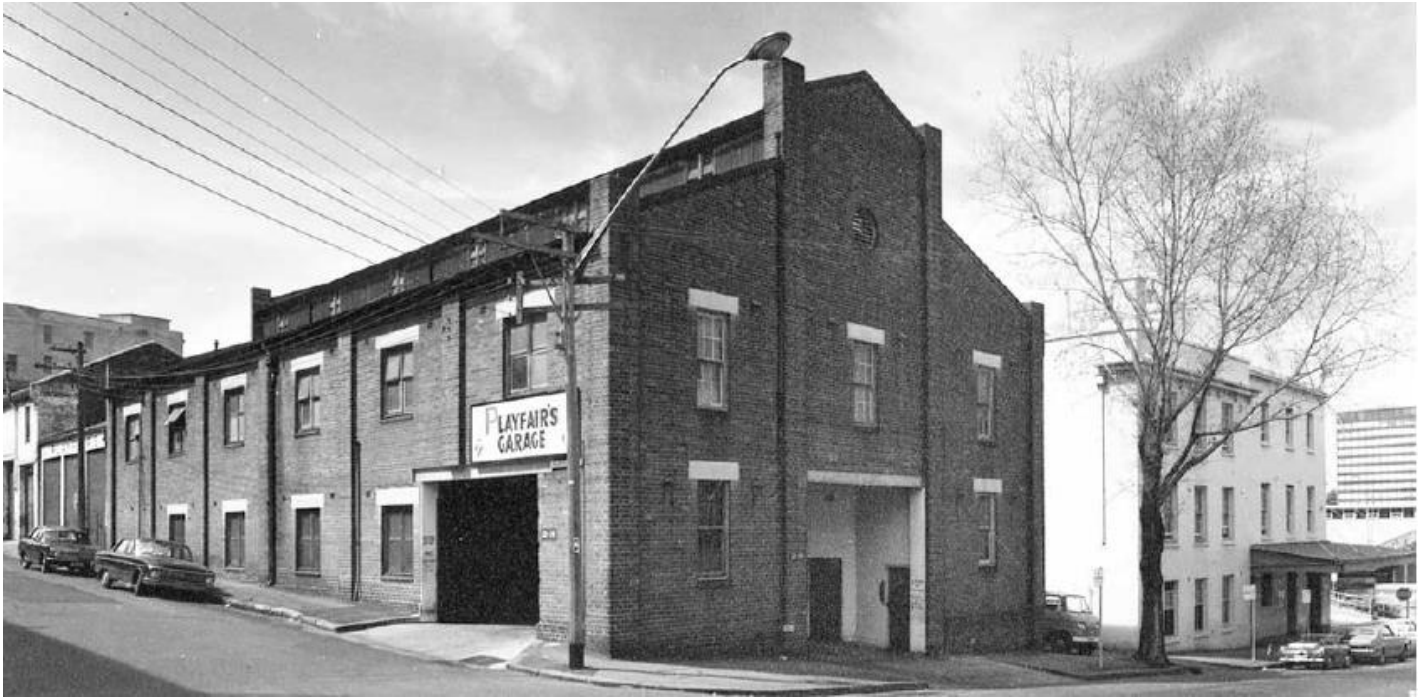
Figure 2.15 Playfair's Garage in 1970. Source: Sydney Harbour Foreshore Authority Archives Image No 40009/742/207
