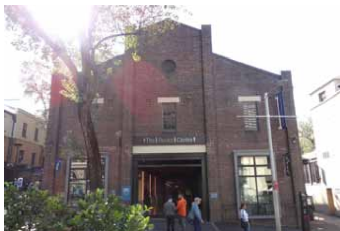
Figure 2.5 Front facade of The Penrhyn House fronting Argyle Street. Note the modified fenestration on the ground floor.
