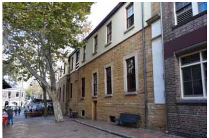
Figure 2.10 The Argyle Stores (former Customs House) houses restaurants and office spaces.
