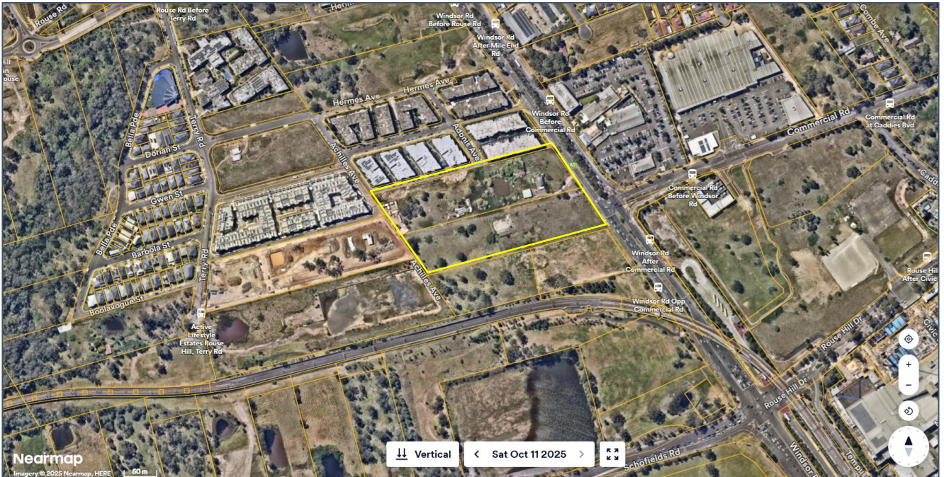
Figure 3 – Aerial view of the site location (Source: Nearmap)
