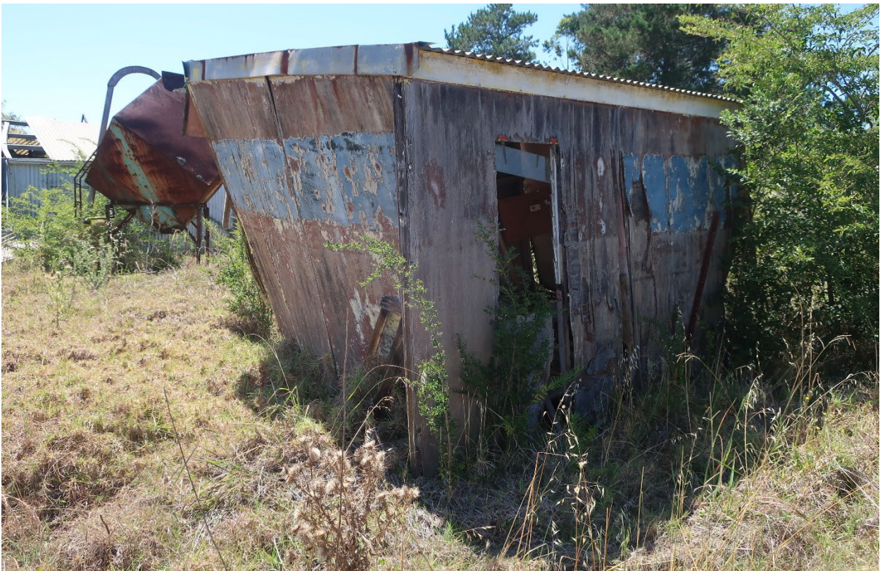
Photo 3-10 A small timber-framed shed west of the larger steel-framed shed
