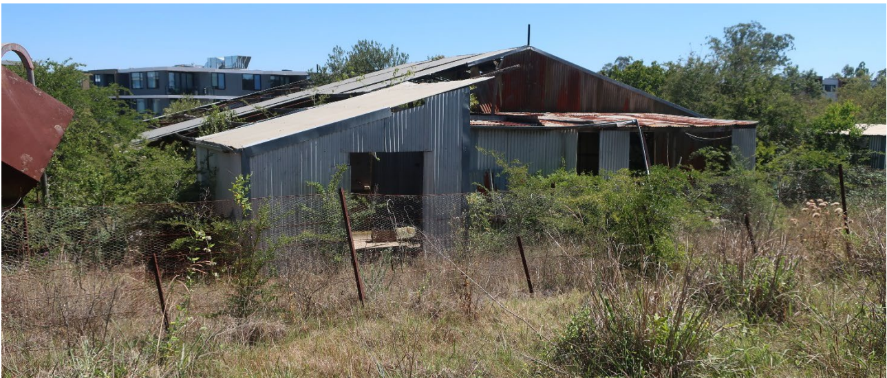
Photo 3-8 A post-war steel-framed shed west of the dam at No. 812
