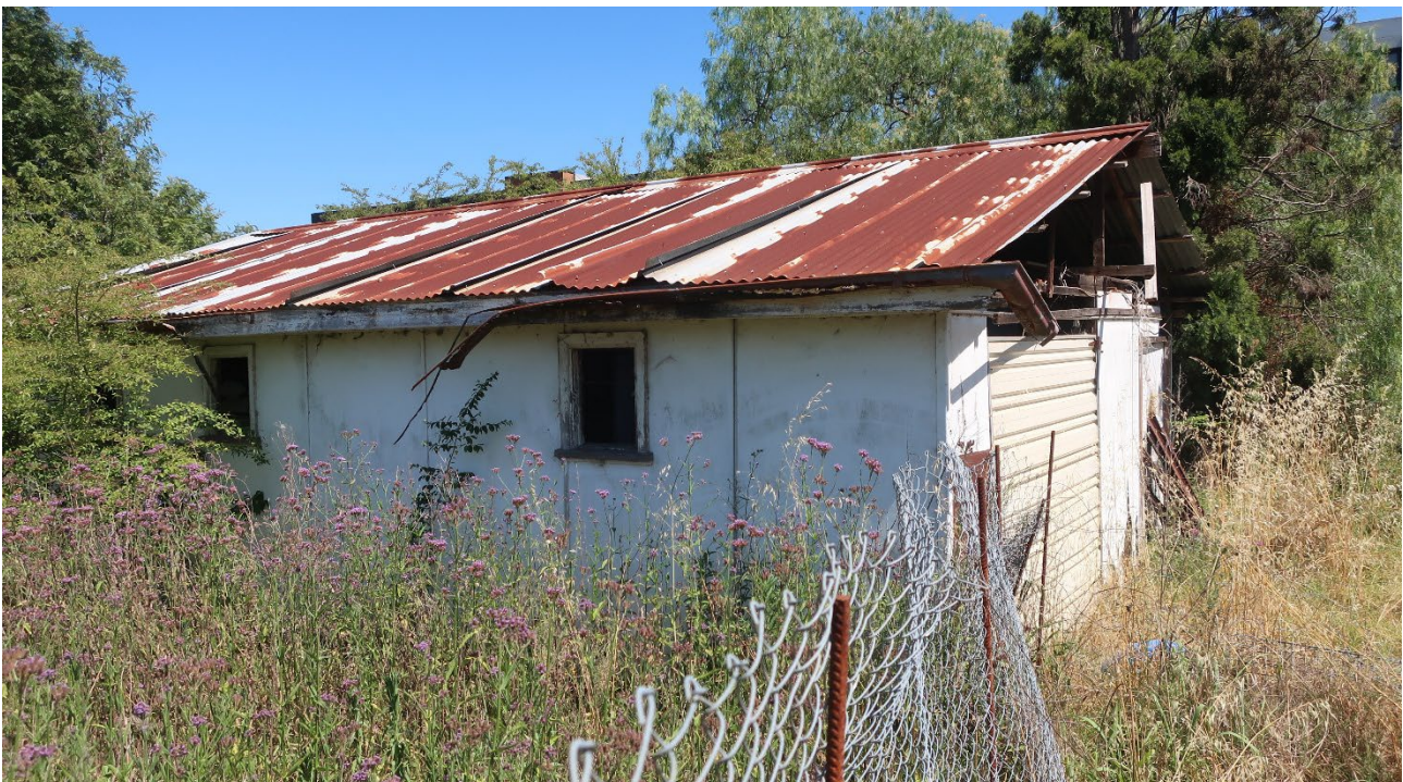
Photo 3-6 Early post-war vehicle shed north-west of the house
