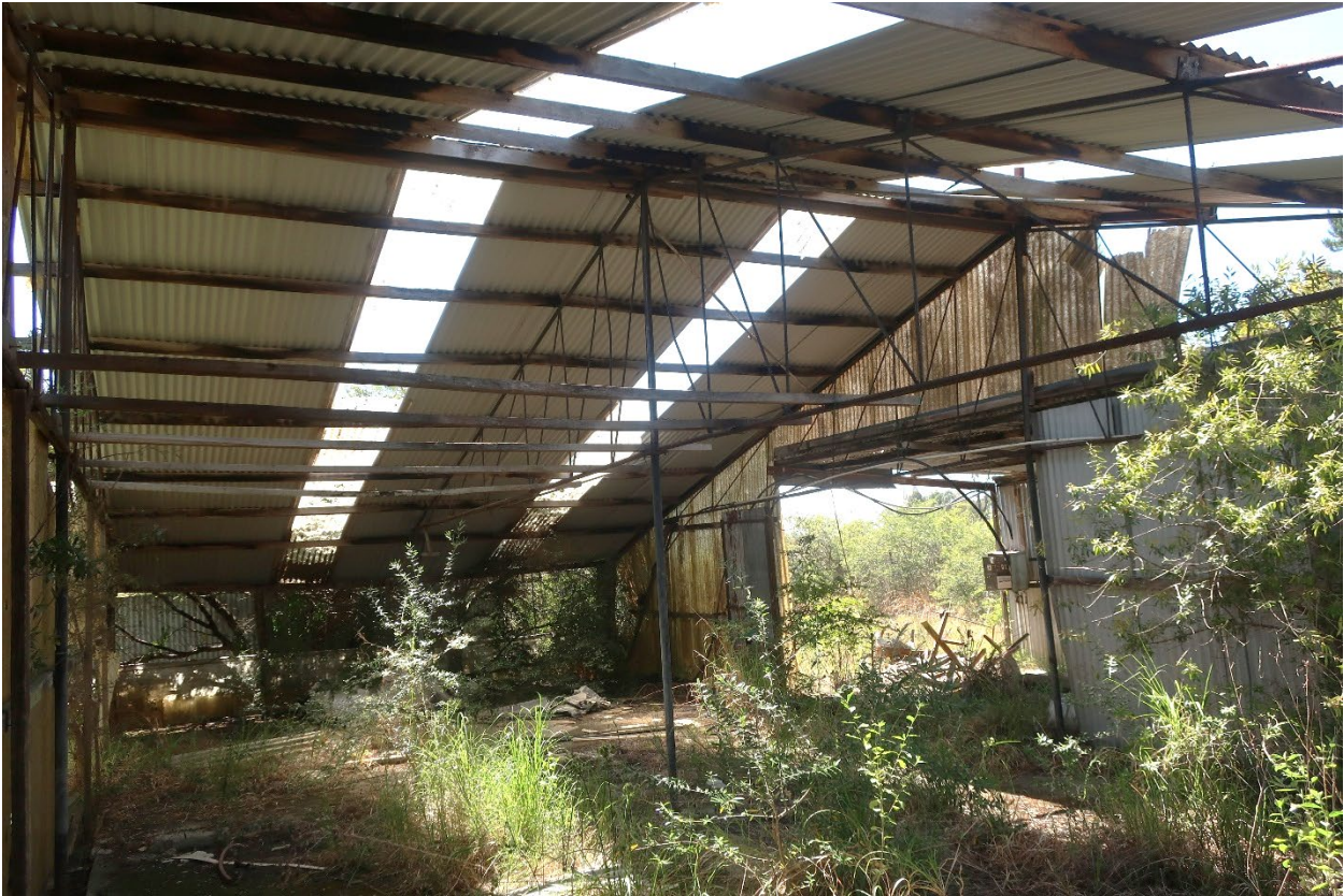
Photo 3-9 Interior of the steel-framed shed, west of the dam at No. 812
