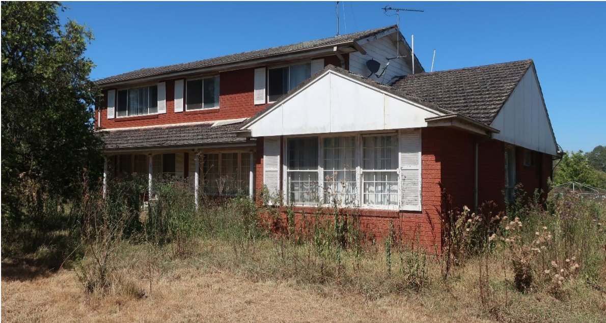
Photo 3-5 The front of the house at 812 Windsor Road
