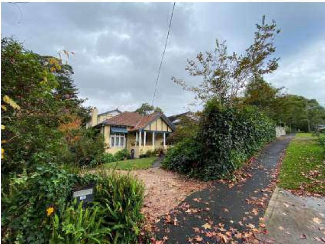
Photograph 12 - Uneven brick and bitumen hard-surfaced area in the front yard were in fair condition (17 Middle Harbour Road)
