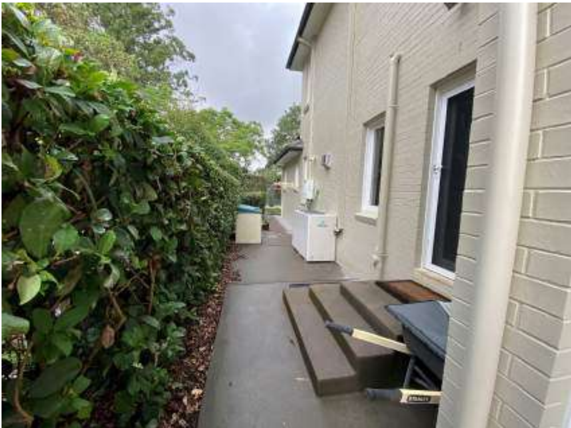
Photograph 10 - The area surrounding the house was surfaced with a concrete slab in good condition (15 Middle Harbour Road)
