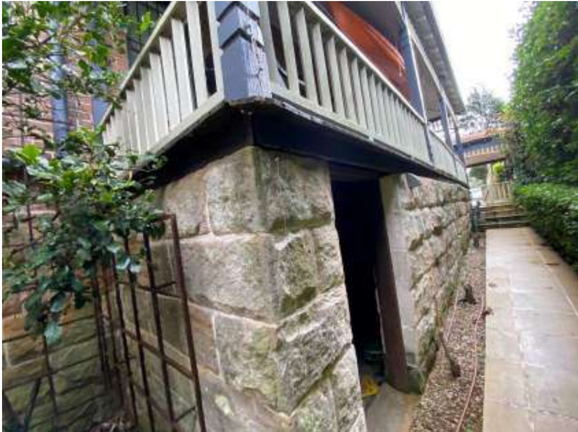
Photograph 3 - Small storage rooms on the lower ground floor (11 Middle Harbour Road)
