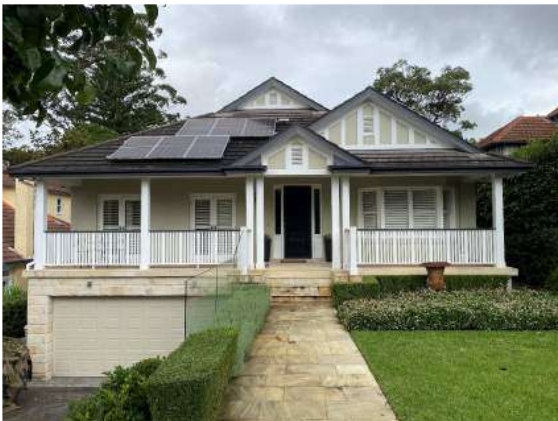
Photograph 6 - Two solar panel were installed on the tiled roof (15 Middle Harbour Road)
