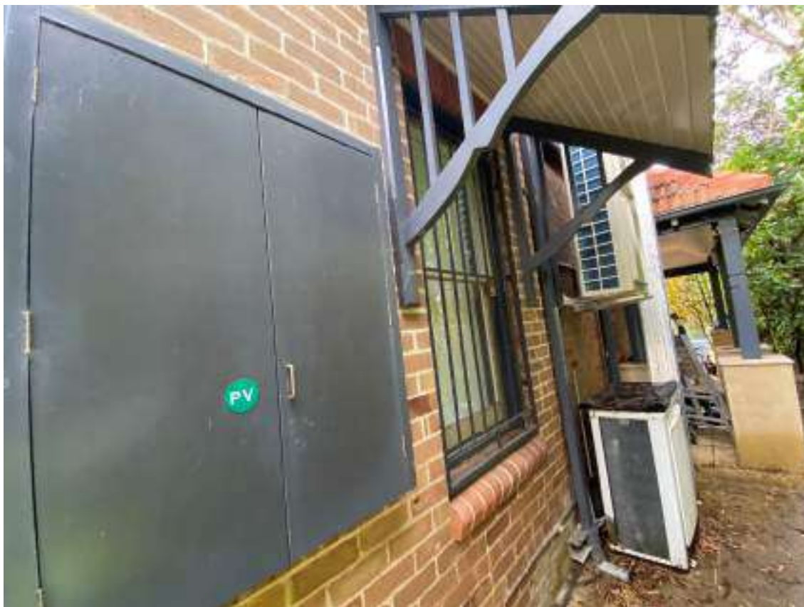
Photograph 5 - An electrical black box and two air conditioning units were mounted on the western wall of the house (11 Middle Harbour Road)
