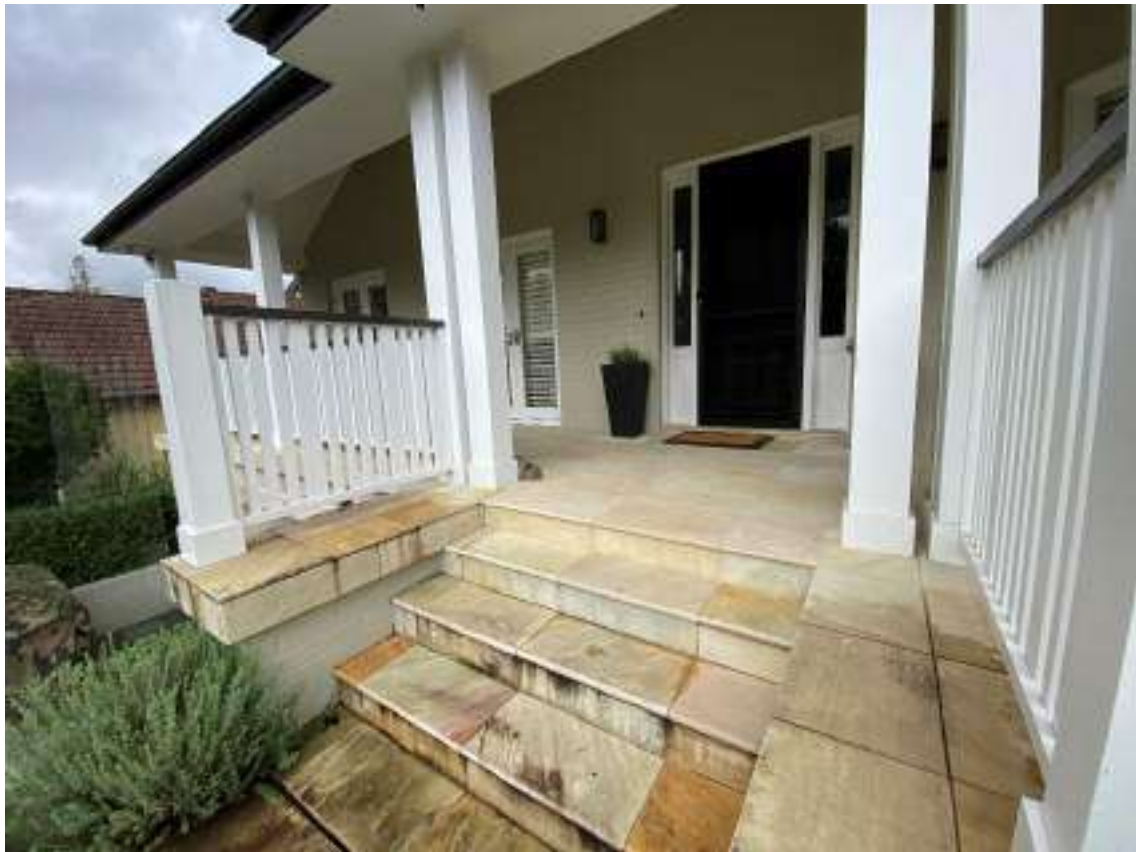
Photograph 11 - Engineered stone was observed around the veranda (15 Middle Harbour Road)
