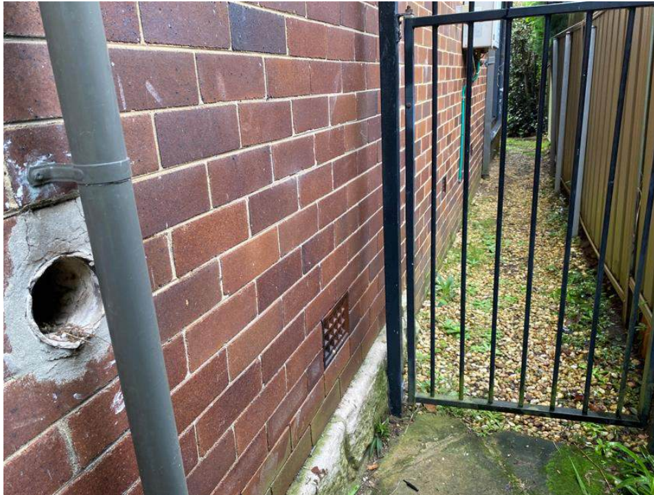
Photograph 7 - 1 Nelson Road - Potential asbestos-containing material (ACM) pipe was found exposed within the brick building on the southern side
