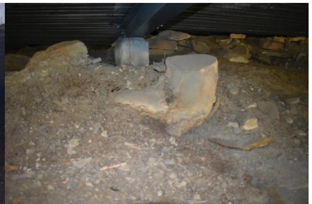
Figure 23: 1 Nelson Road, tree stump on fill beneath tennis court platform
