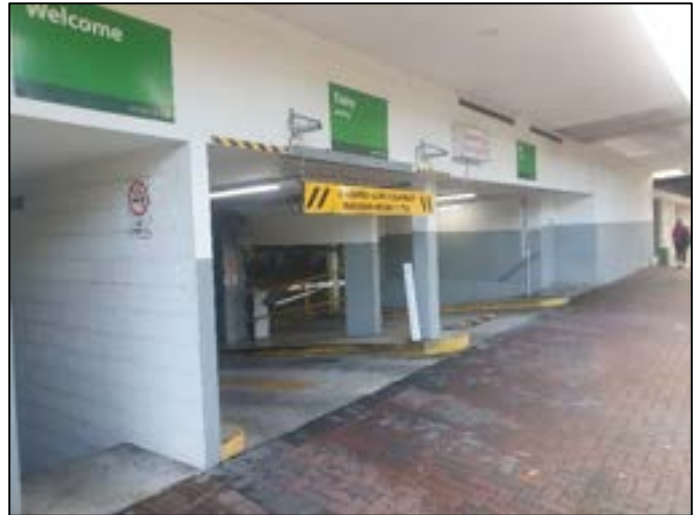
Plate 10 – Underground carpark entrance from Yeo Street.
