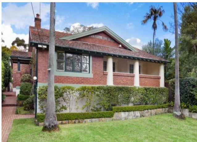
Figure 4 The front facade of 28 Bent Street, Lindfield (I416) Source: NSW Heritage Inventory
