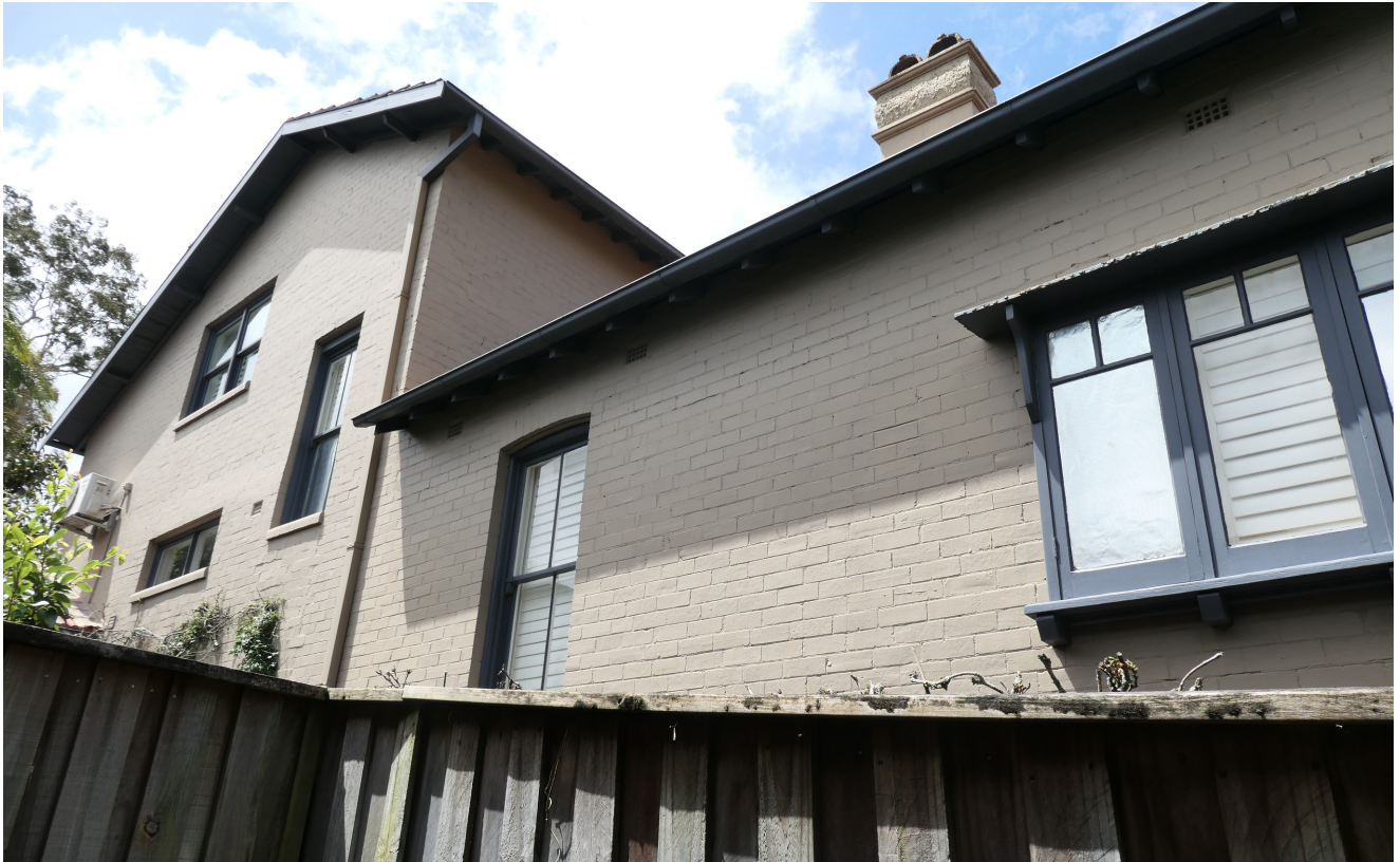
Figure 23 21 Balfour Street: the side elevation with 1988 additions
