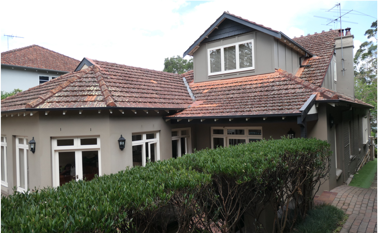
Figure 14 The rear and side elevations of 19 Balfour Street
