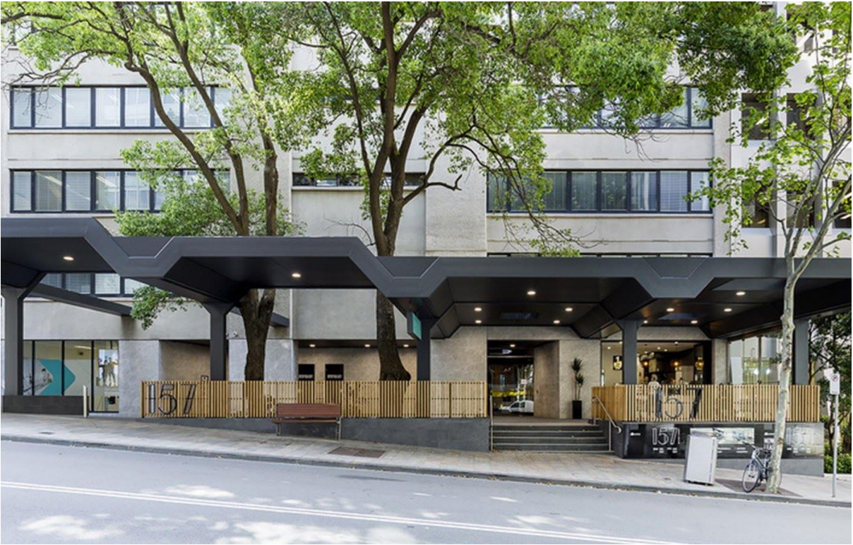
Existing 153 - 157 Walker Street Entrance
