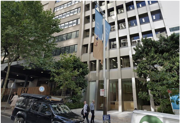
153 - 157 Site from Walker Street South
