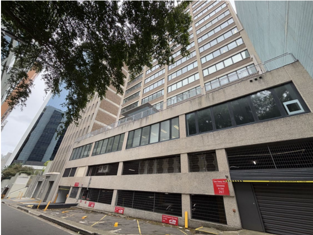
Figure 3 Little Walker Street looking towards rear of 157 Walker Street
