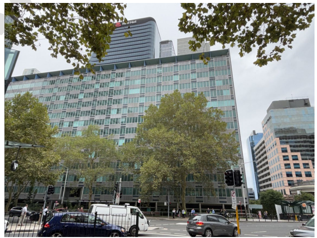
Figure 29 MLC Building, 205-153 Walker Street, North Sydney
