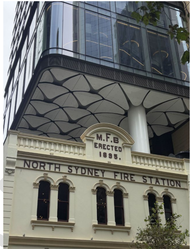
Figure 10 Close up of Former Fire Station from Walker Street
