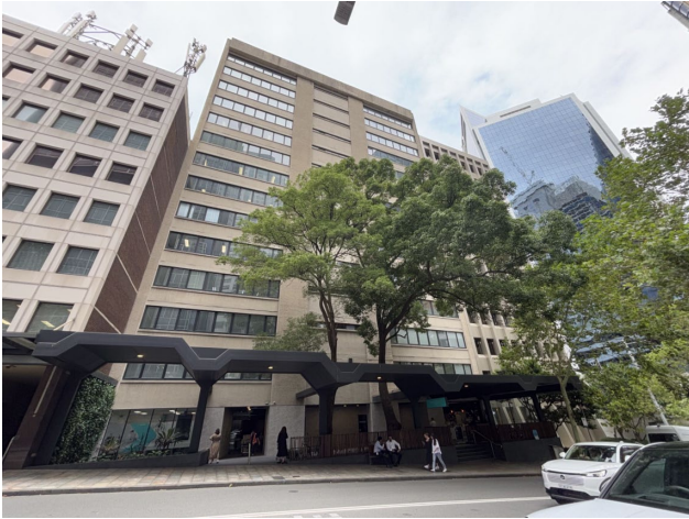
Figure 13 157 Walker Street primary concrete-rendered façade with protruding marquee.
