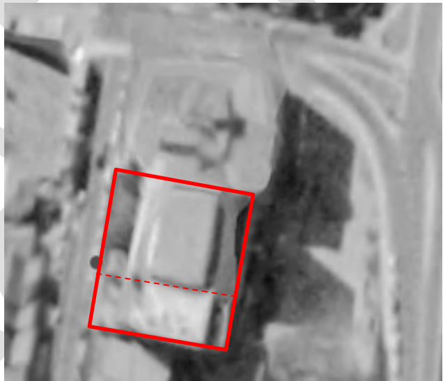
Figure 22 1970 imagery indicating construction of present high-rise towers at 153-157 Walker Street
