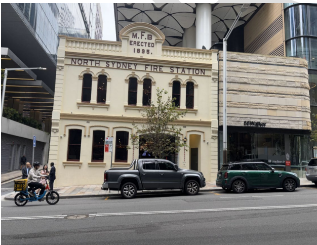
Figure 28 Former Fire State, 86 Walker Street, North Sydney
