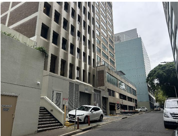
Picture 3 View of rear entrance to 153 Walker Street (left) and 157 Walker Street (right) from Little Walker Street
