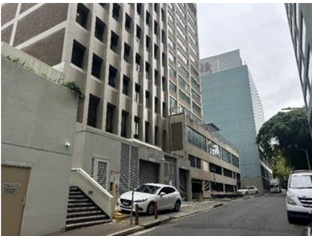
Picture 3 View of rear entrance to 153 Walker Street (left) and 157 Walker Street (right) from Little Walker Street
