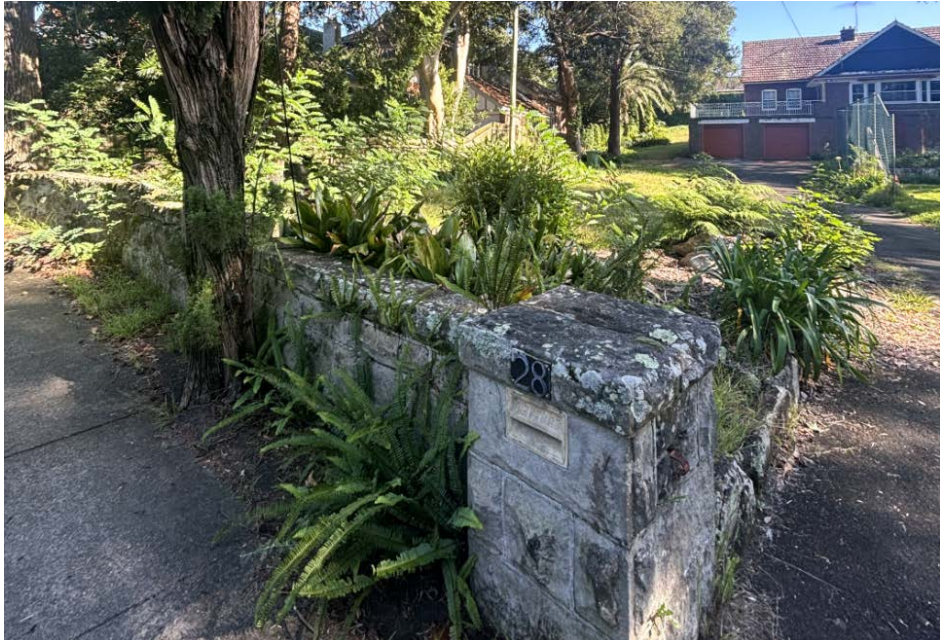
③ Existing Sandstone walls and frontages
