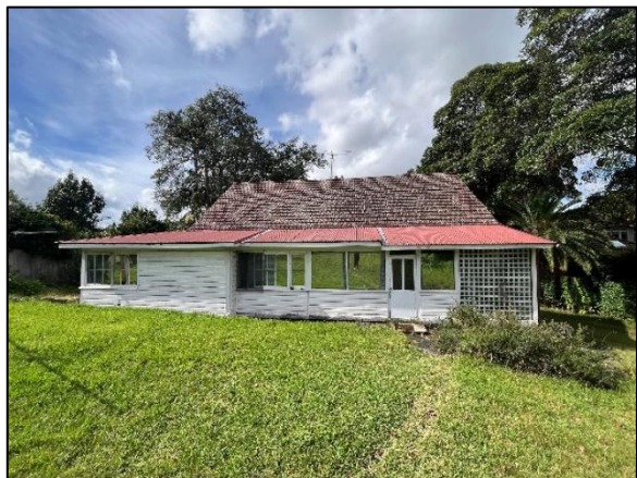
Figure 40. Rear weatherboard addition with corrugated metal roof sheeting. Facing south.
