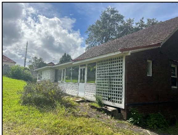
Figure 39. The rear of the dwelling with late-addition weatherboard and corrugated iron roof sheeting. Facing south-east.
