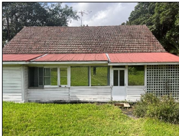
Figure 41. Close up of contemporary materials and windows. Facing south.
