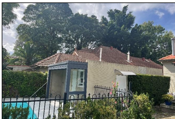
Figure 70. Facing south-east to contemporary garage.
