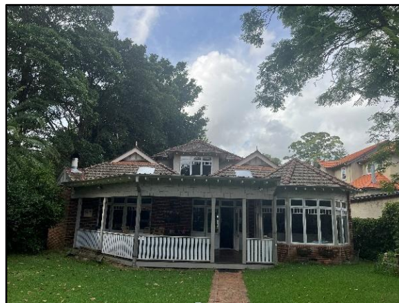
Figure 57. The rear of 26 Middle Harbour Road with contemporary rear addition and second-storey addition. Facing south-east.
