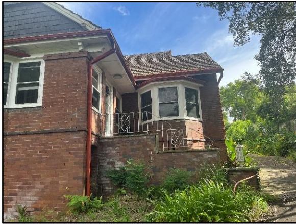
Figure 44. Facing north to part of the primary (southern) façade.
