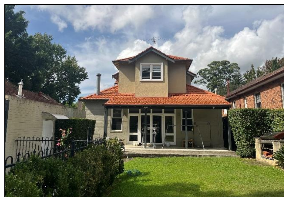
Figure 71. Facing south to modified rear of dwelling.
