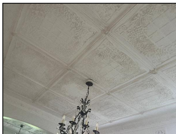
Figure 65. Internal view of original ornate fibre plaster ceilings at 24 Middle Harbour Road.
